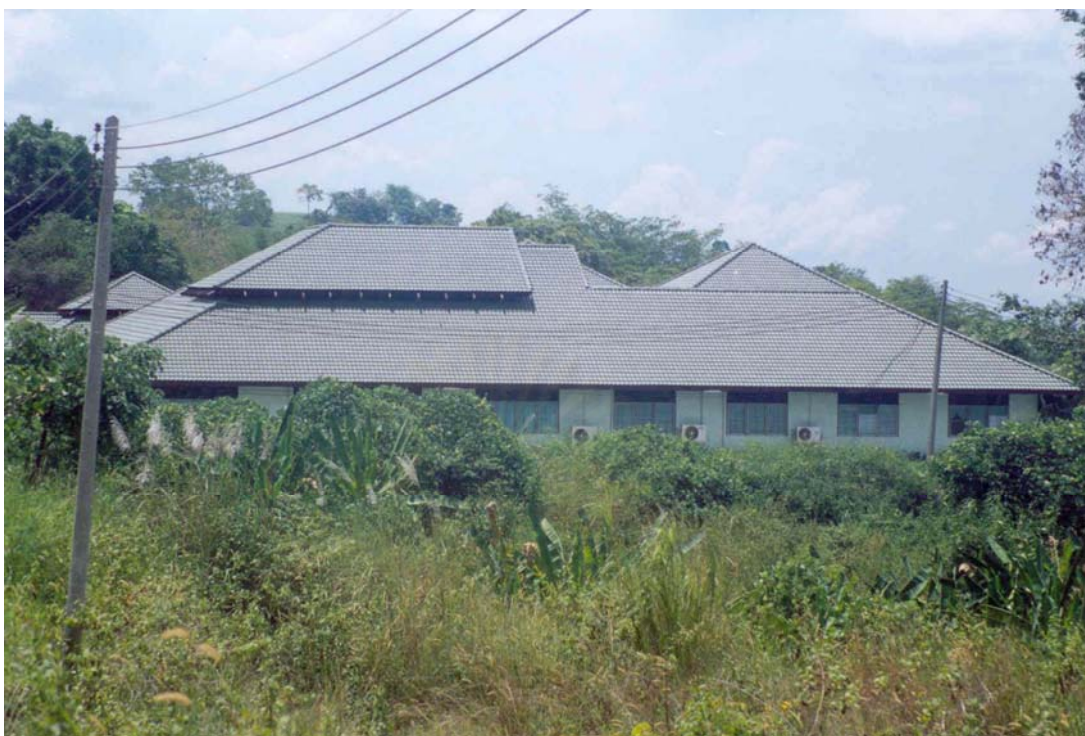
Figure 3-4 The residential complex in Khao-Khiao Open Zoo, Khao Khiao–Khao Chomphu Wildlife Sanctuary, Chon Buri Province
