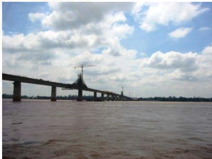
Construction Site of Second Mekong International Bridge
