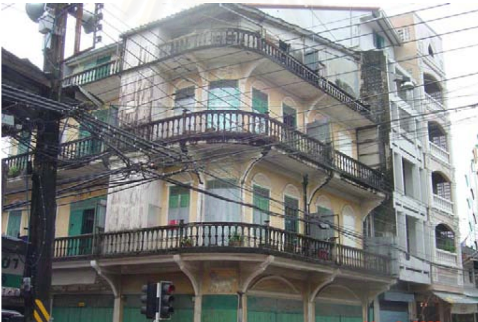
Figure 4.6. An old building modified for A. fuciphagus at Pak Phanang District, Nakhon Si Thammarat Province.
