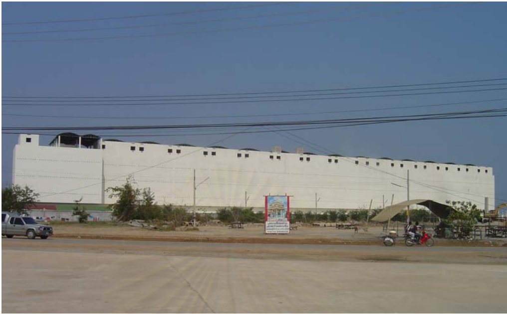
Figure 4.5. A newly constructed building for swiftlets located at Ban Leam District, Petchburi Province.
