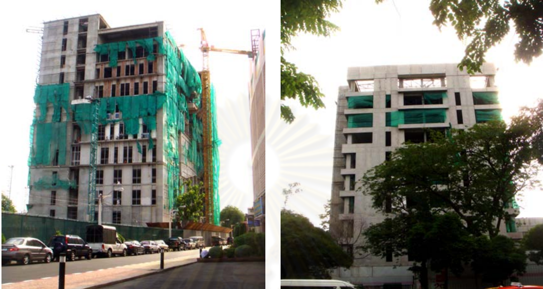
Figure 4.14 Pictures of surveyed construction sites in Thailand
