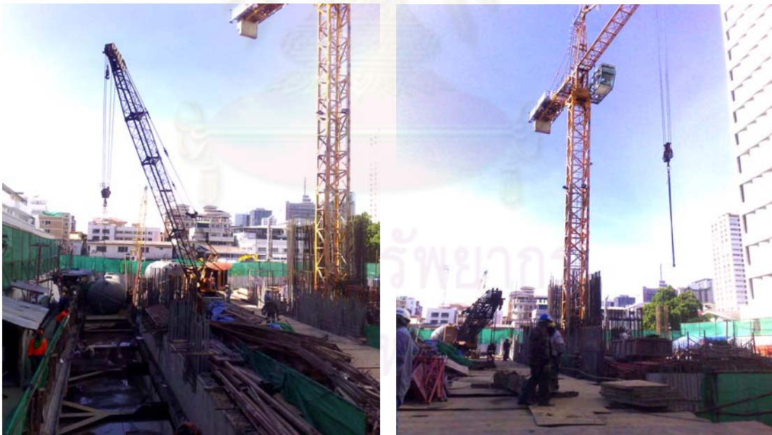
Figure 4.14 Pictures of surveyed construction sites in Thailand
