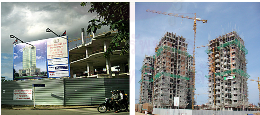
Figure 4.8 Building projects under construction in Phnom Penh
