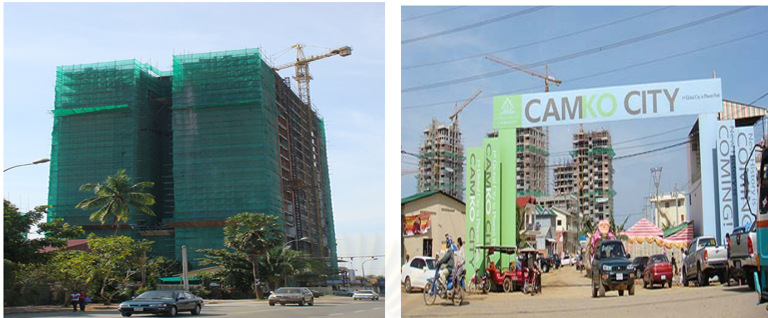
Figure 4.8 Building projects under construction in Phnom Penh
