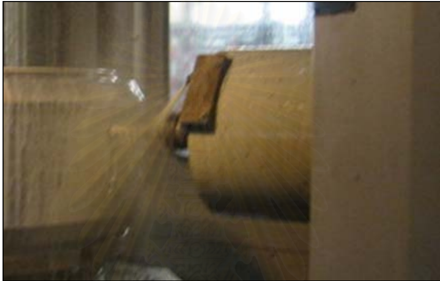
Figure 6.10 : New Drill During Work
