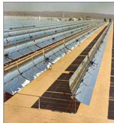
Figure 1.10 Schematic diagram of parabolic trough system
