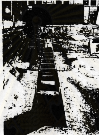
CAST IN PLACE PRETENCH
