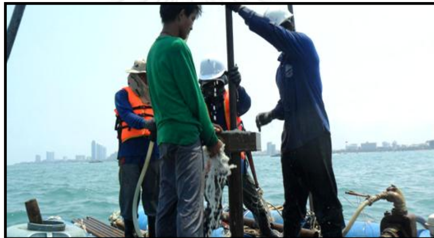
Figure 28 Counter flush reverse circulation.
