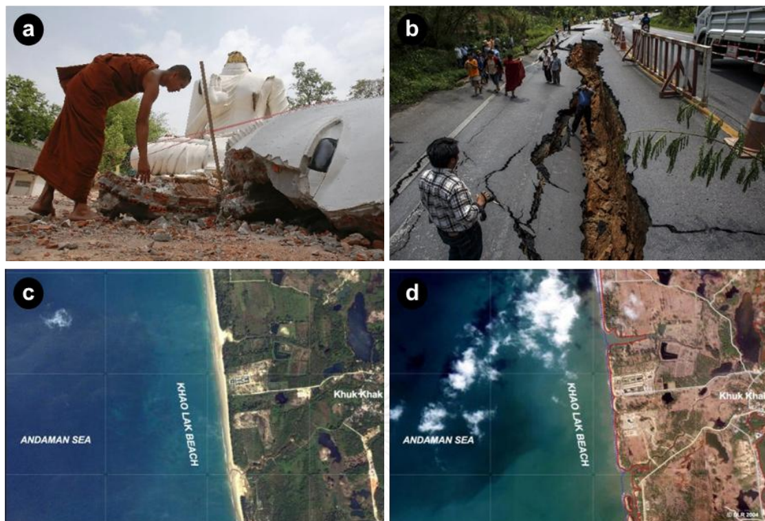
Figure 1.3. a) A severely damaged Buddha statue in the Udomwaree temple, Chiang Rai, Thailand, after the occurrence of the M_w -6.2 Mae Lao Earthquake on May 5, 2014 (Chiangrai Times, 2014). b) The a large crack (over 50 meters stretch) on the highway No. 118 around kilometer marker 141, between Mae Lao and Mae Sruay districts, Thailand (Perawongmetha, 2014). c and d) Khao Lak beach before and after the M_w -9.0 Sumatra-Andaman earthquake on December 24, 2004, respectively (Jarl, 2005).
