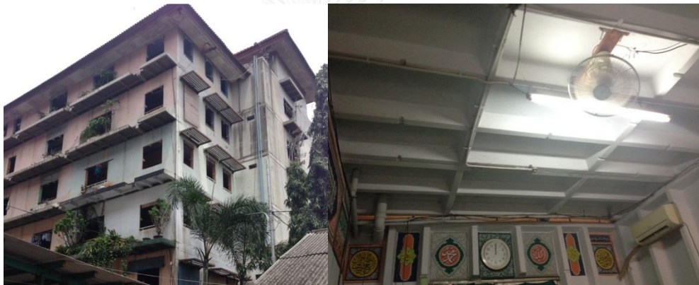
(a) Exterior of waffle-crete system (b) Interior of waffle-crete system
