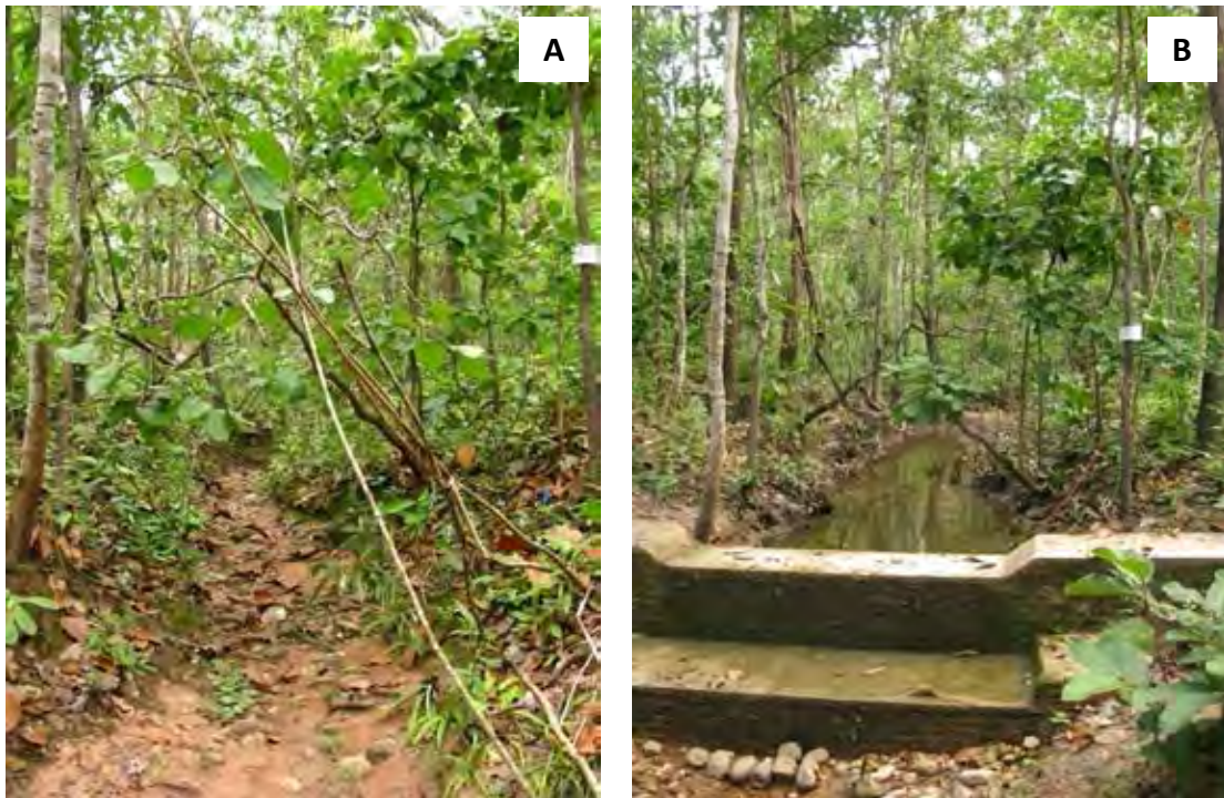
Figure 3-5 Photographs of the stream B between pre- and post-check dam periods. The letter A and B indicated pre- and post-check dam periods, respectively.
