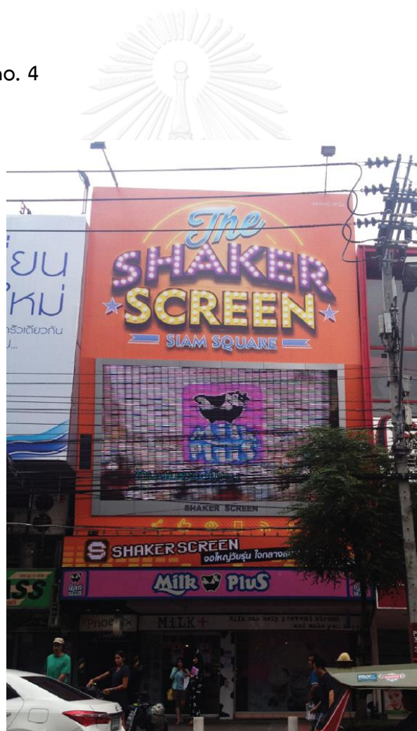
Figure 24 Shophouse frontage no.4
