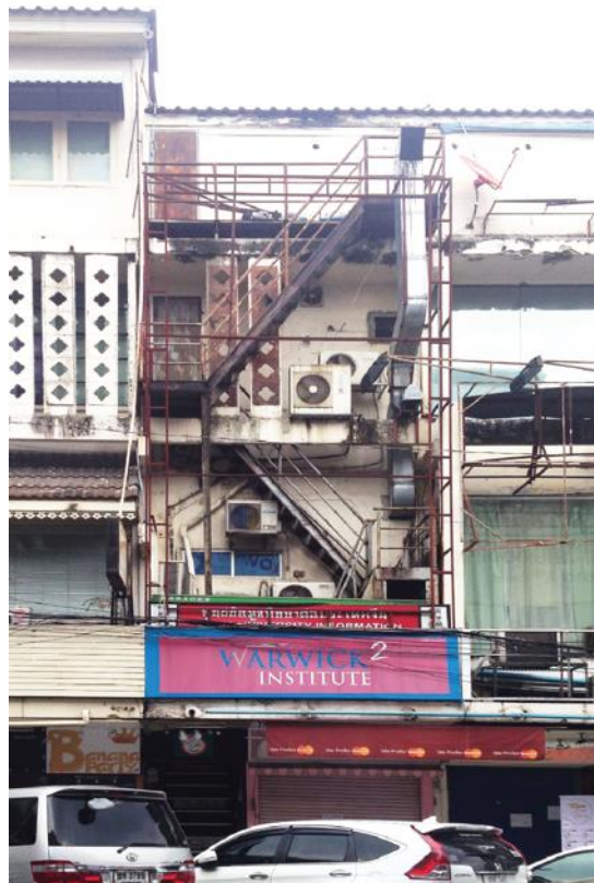
Figure 22 Shophouse frontage no.3
