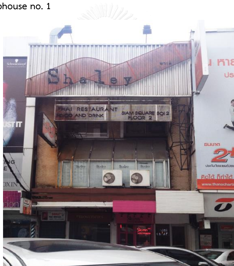
Figure 18 Shophouse frontage no.1
