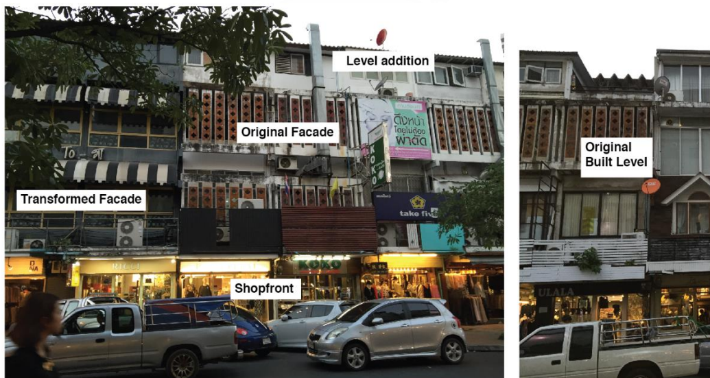
Figure 16 Shophouse transformation in Siam Square
