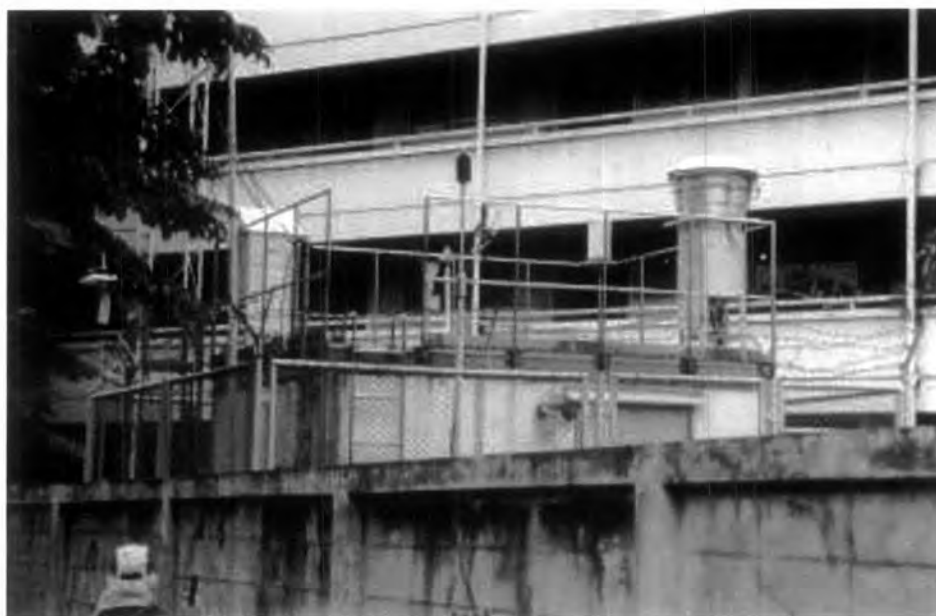
Figure 3.2: Ladphrao monitoring station
