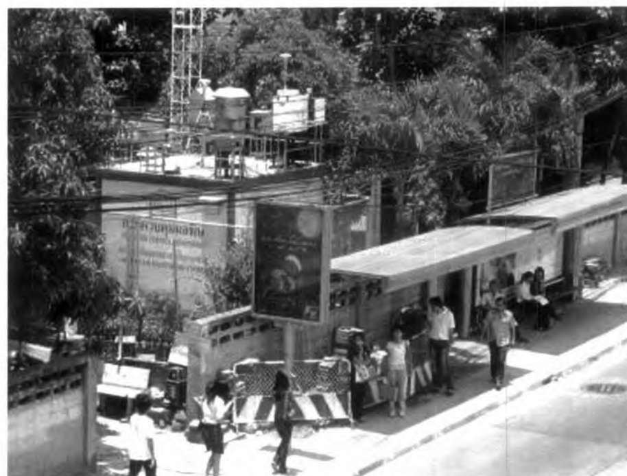
Figure 3.4: Dindaeng monitoring station
