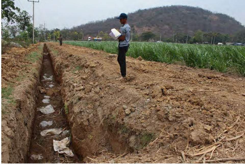
Station 4: Trench near 324 road
