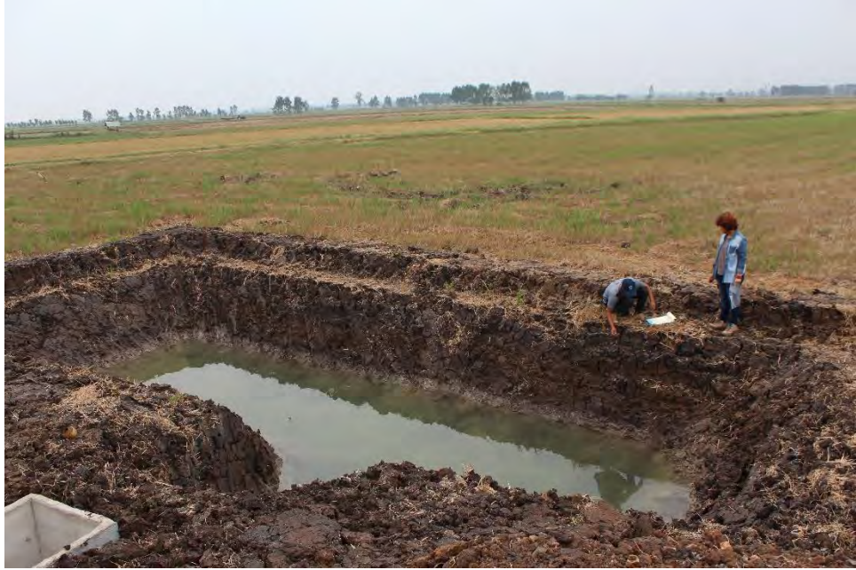
Station 11: Unit H
