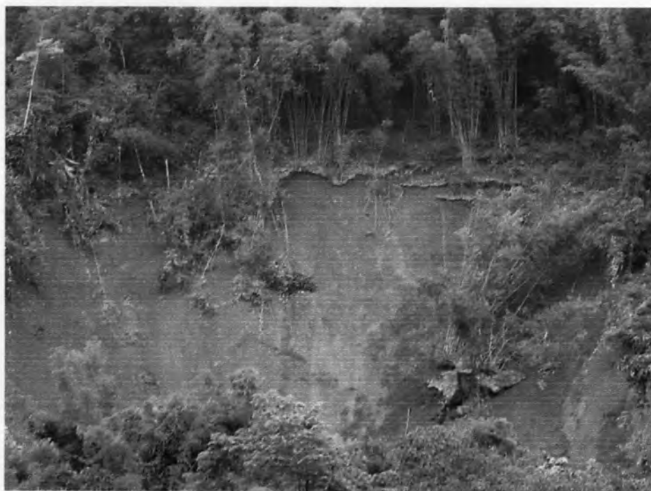
Figure 4.1 Shallow landslide of weathered surface at Nam Phoe Village, Thung Chang District, Nan Province.
