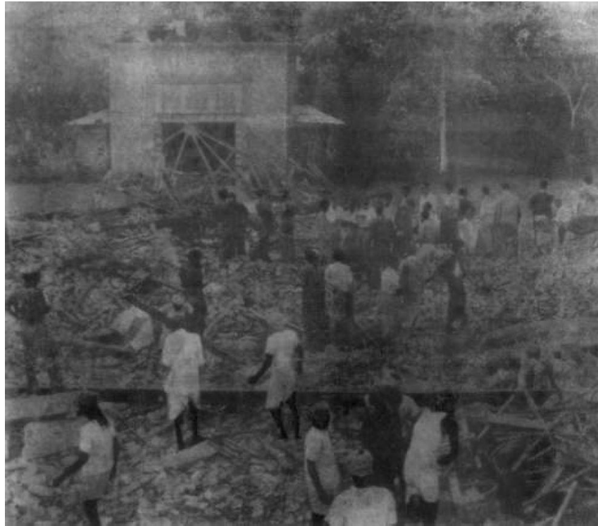
Figure 4. 8. Student Union after it was demolished (July 1962).
