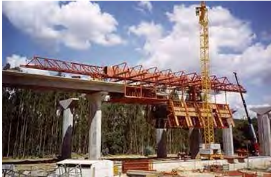
Figure 4.6: The MSS Movable Formwork System Source: www.Structurerae.com
