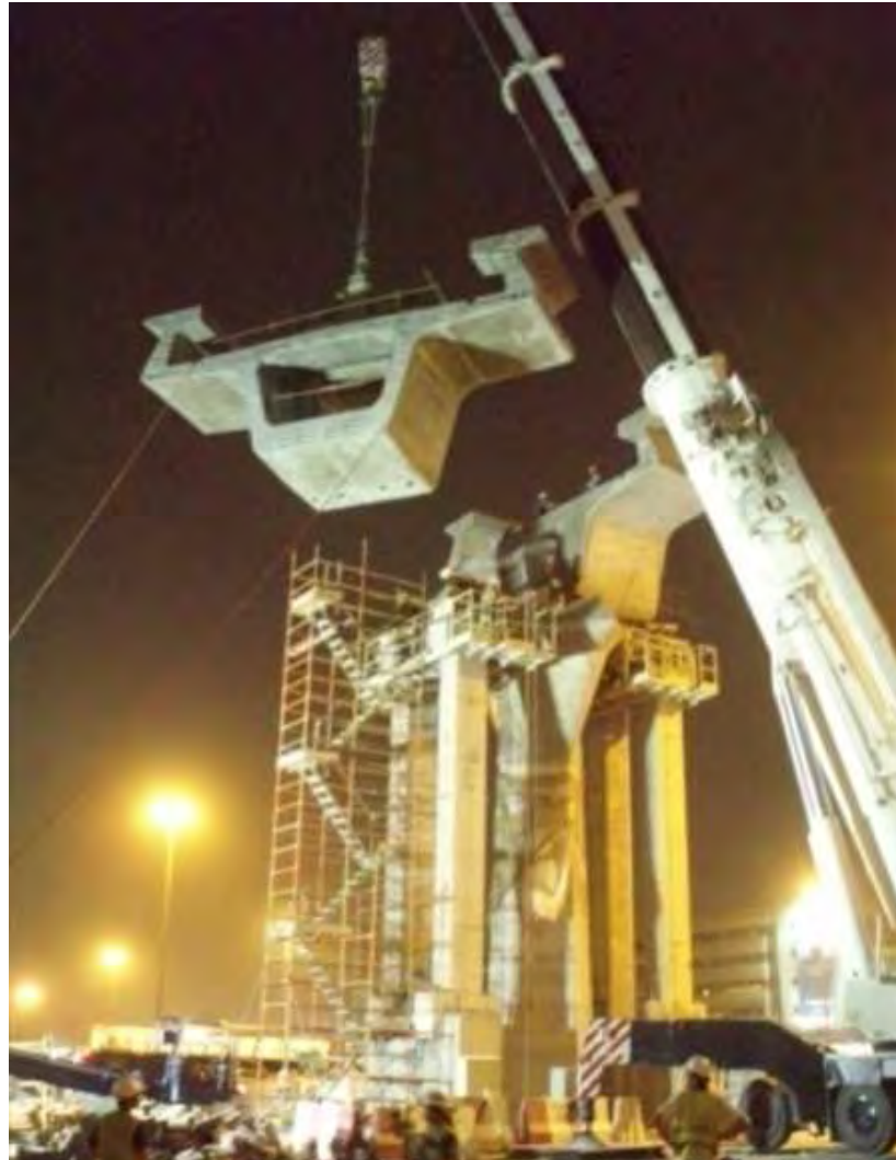
Figure 4.15: Pier Head Segments are Erected by Crane Source: www.launching-gantry-operator.com
