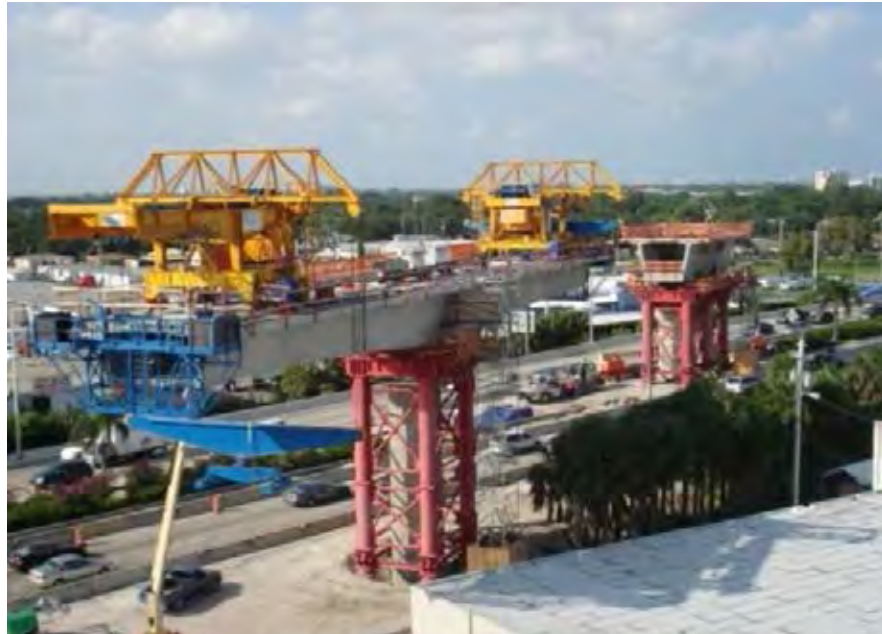
Figure 4.14: Lifting Both Segments Using a Lifting Frame Source: www.launching-gantry-operator.com
