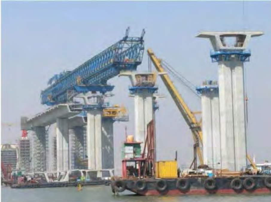
Figure 4.13: Balanced Cantilever by Launching Gantry Source: www.launching-gantry-operator.com
