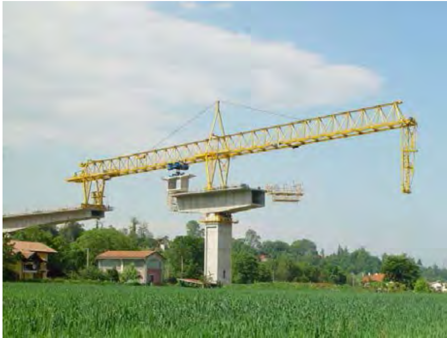
Figure 4.12: Balanced Cantilever Bridge
