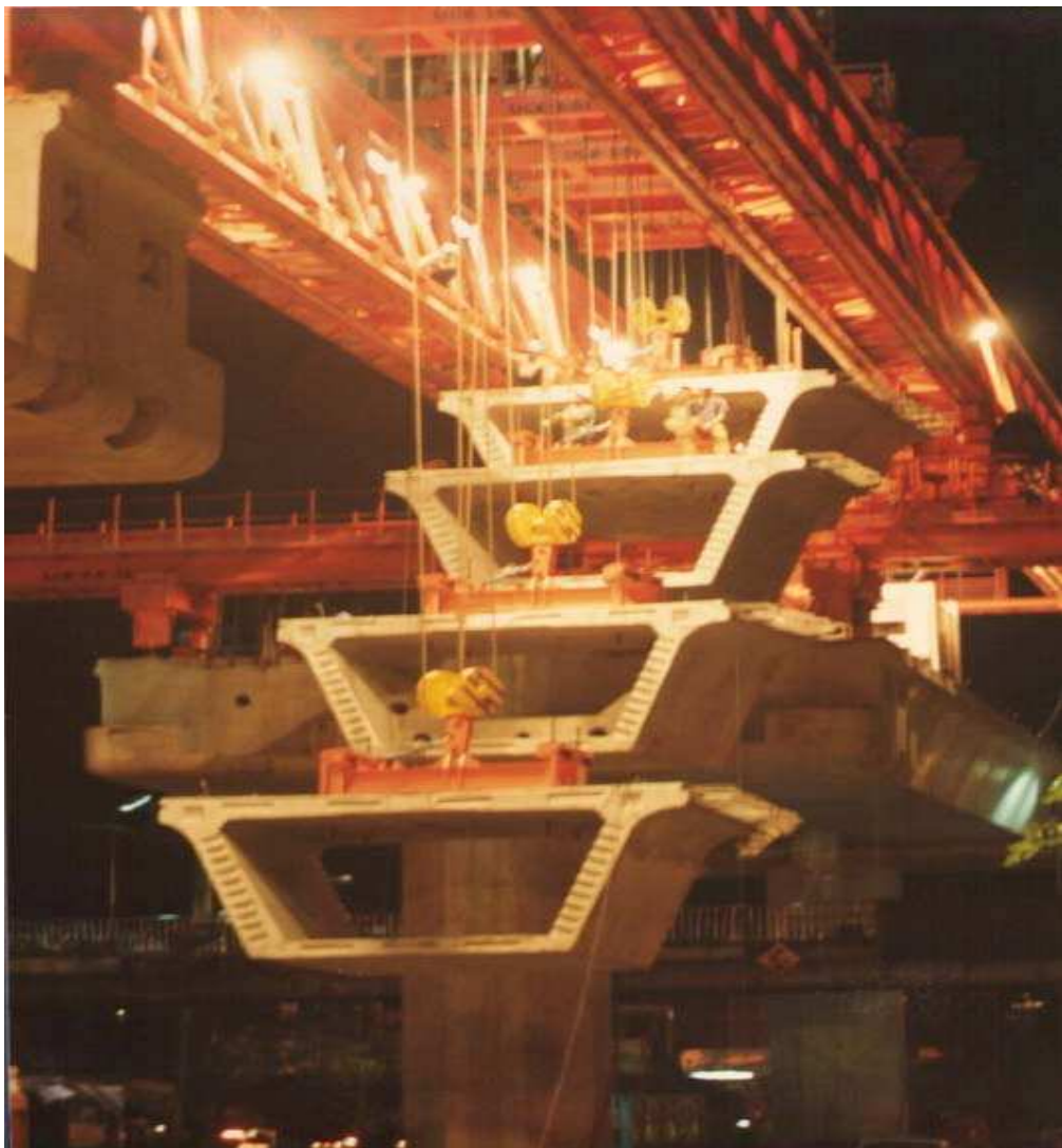
Figure 4.1: Concrete Box Segment Source: IABSE, (2011)
