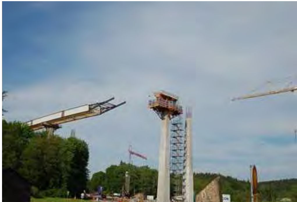
Figure 4.4: Incremental Launching Method: Amal Motorway Bridge, Sweden. Source: www.Structurerae.com
