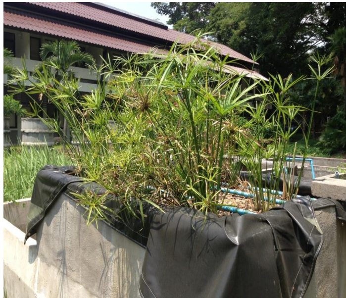
Figure 3.1 The VF CW system
