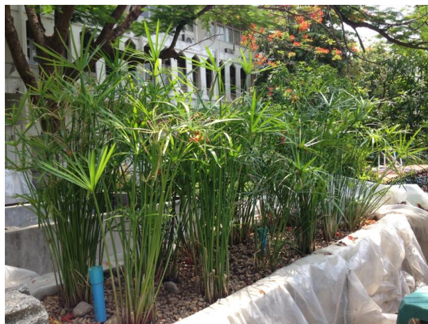
Figure 3.3 The HSSF CW system
