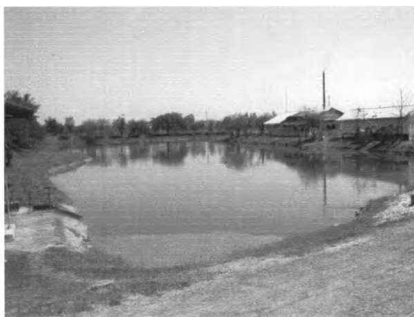
Figure 3.1 Final polishing pond of the central wastewater treatment plant of the Northern Region Industrial Estate
