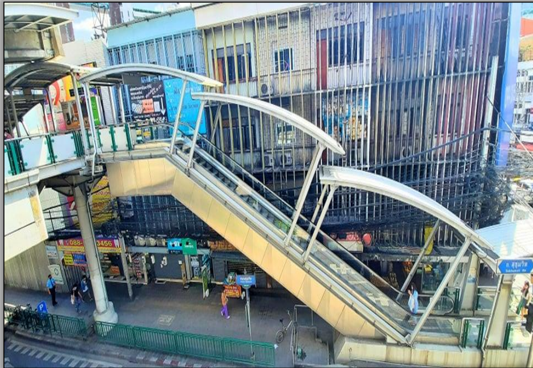
Poor visibility of the business on the ground floor & lack of privacy in the upper floors are created by BTS line
