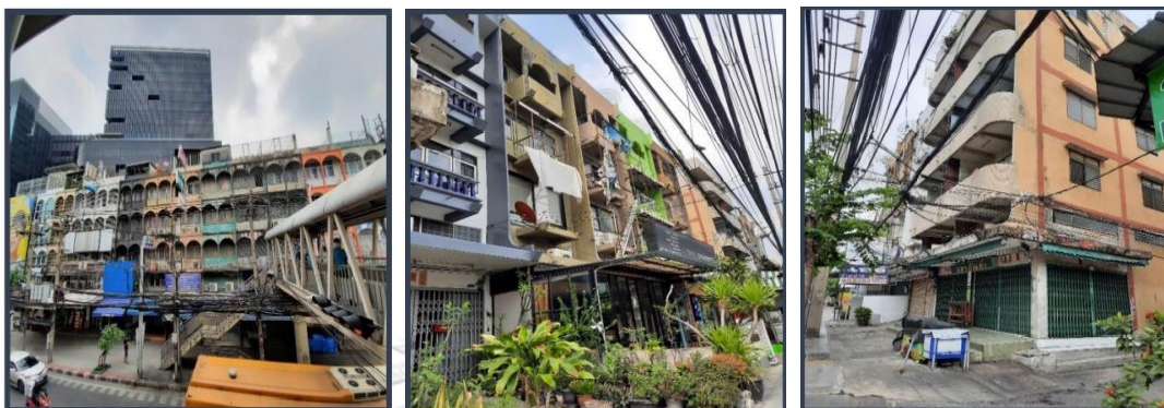
Figure 1: Shophouse buildings in Punnawithi area
