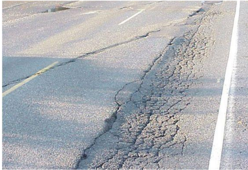
Figure 2.11 Rutting deformation [67]
