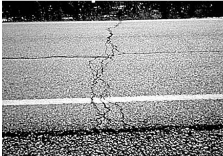
Figure 2.12 Thermal cracking [67]
