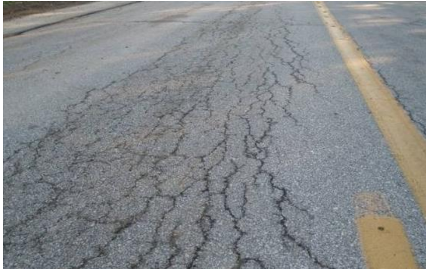
Figure 2.13 Fatigue cracking [67]
