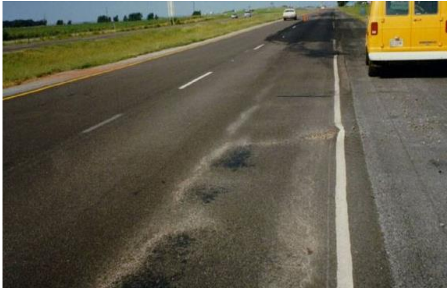
Figure 2.14 Moisture damage [67]
