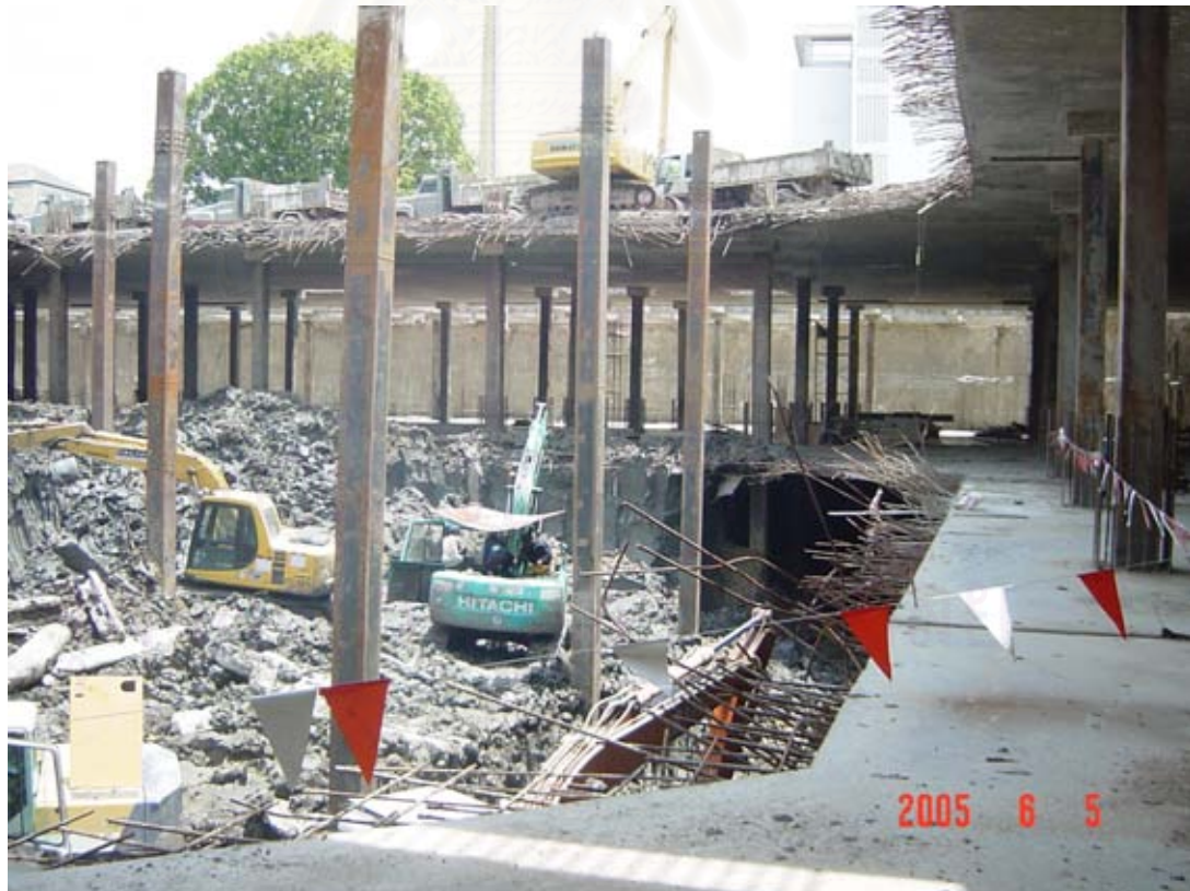
Figure 3.8. BOT project under construction
