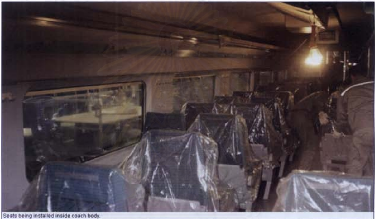
Seats being installed inside coach body.
