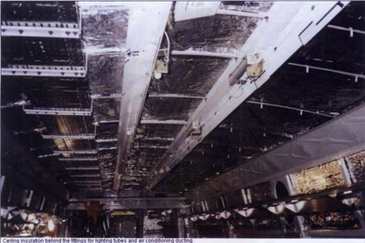
Ceiling insulation behind the fittings for lighting tubes and air conditioning ducting
