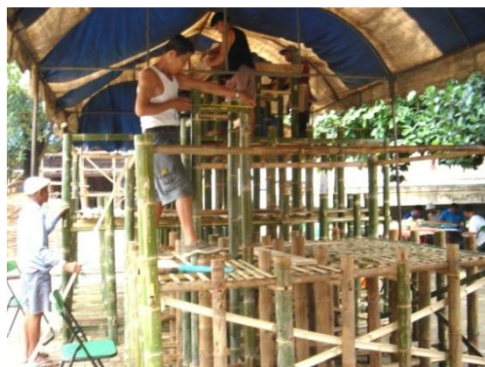
Figure 53 Constructing the base with Phai Si Suk bamboos
