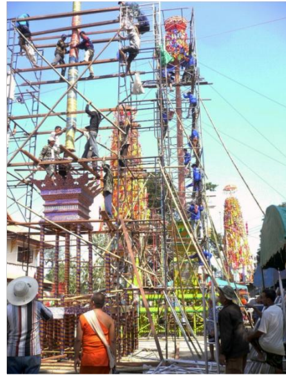
Figure 56 Securing the pole Source: SP
