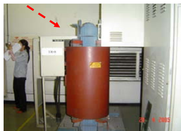
Existing TR at Substation Rm. 19 th FL. To be demolished (TR7,8 @ 1000KVA)
