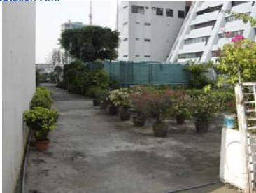
This Area at 8 th Floor to be Renovated to new Substation Rm.
