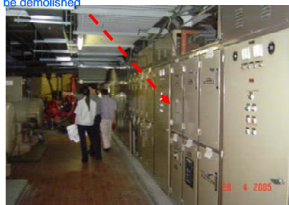
Existing EMP Panel at Generator Rm. B FL. To be demolished
