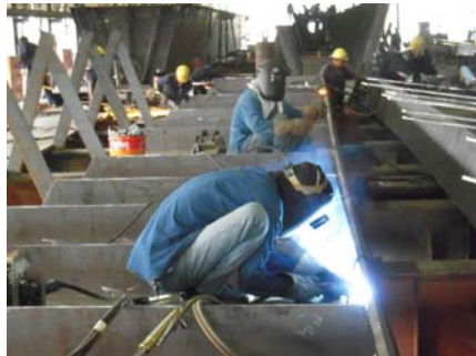
Figure 4.13b Stiffener and web flange welding
