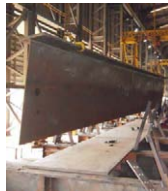
Figure 4.12d Box girder assembling
