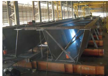
Figure 4.13c Box girder welding
