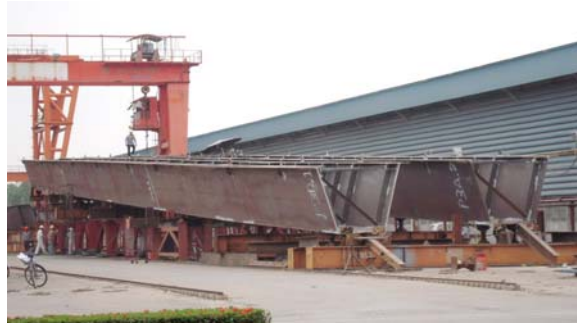
Figure 4.6 Trial assembly of three span length box girders
