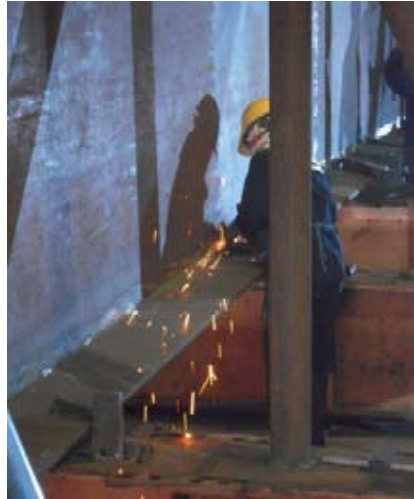
Figure 4.13a Web and top flange welding
