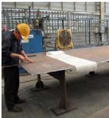
Figure 4.10a Drilling template preparations
