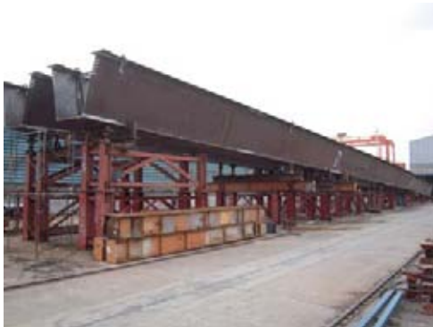
Figure 4.15c Three pairs of box girders
