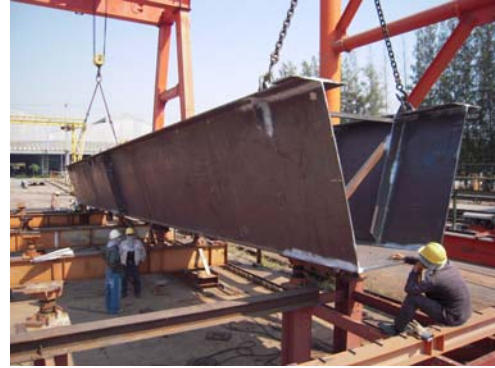
Figure 4.15b Trial assembly activity
