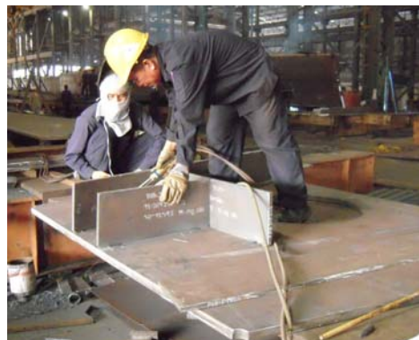
Figure 4.12c Diaphragm assembling
