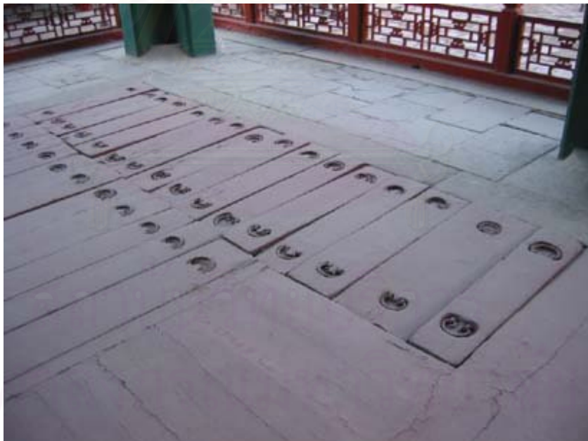
Pic. 15 b. The pathway to the underground covered with the “movable covered boards” on the Longevity Stage. Photo taken inside the Longevity Stage of the Pleasant Sound Pavilion by Sasiporn Petcharapiruch on November 11, 2004.
