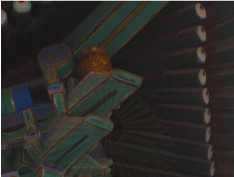
Pic. 19 c. The close-up view of the cantilevered arms ( ang 昂) in the east side of the three-tiered stage the Pleasant Sound Pavilion. Photo taken by Sasiporn Petcharapiruch on November 11, 2004.
