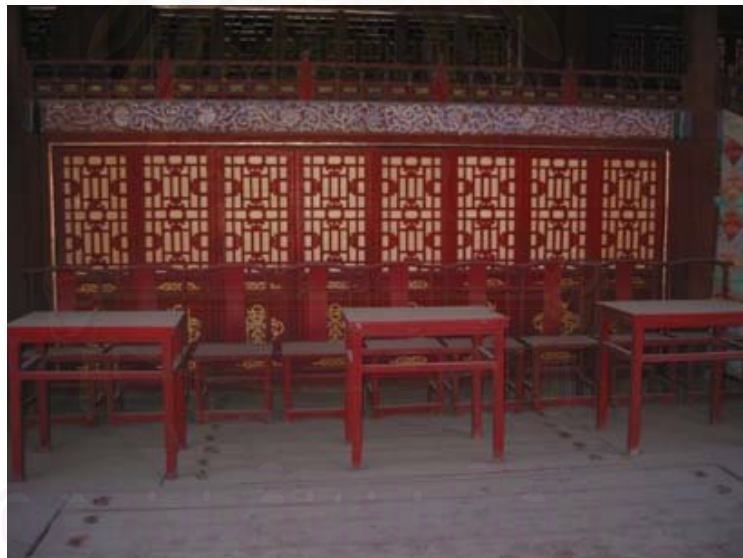
Pic. 9. Screen doors ( gezimen 格子門) between the front stage and the backstage of the Longevity Stage, connected to the Immortal Tower. Photo taken inside the Longevity Stage of the Pleasant Sound Pavilion by Sasiporn Petcharapiruch on November 11, 2004.
