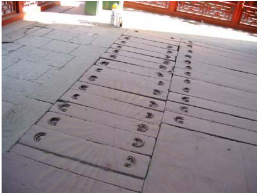
Pic. 15 a. The pathway to the underground area covered with the “movable covered boards” on the Longevity Stage. Photo taken inside the Longevity Stage of the Pleasant Sound Pavilion by Sasiporn Petcharapiruch on November 11, 2004.
