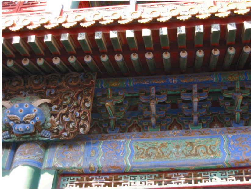
Pic. 19 a. The bracketing system in the east side of the three-tiered stage the Pleasant Sound Pavilion. Photo taken by Sasiporn Petcharapiruch on November 11, 2004.
