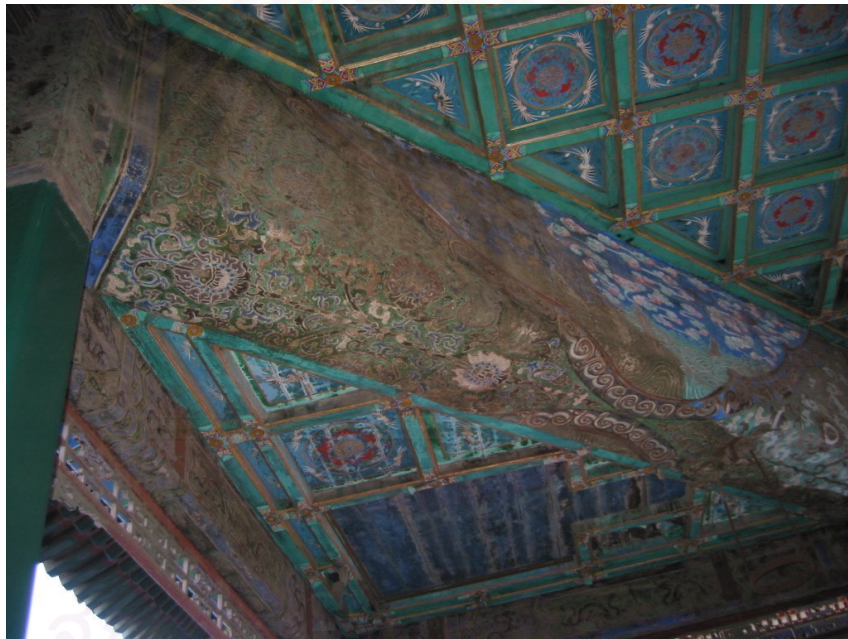
Pic. 33 b. The Suzhou style of multicolored oil painting on the corner girder of the inner eave in the Longevity Stage. Photo taken by Sasiporn Petcharapiruch on November 11, 2004.
