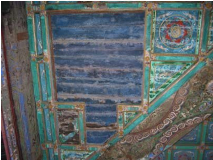
Pic. 13 b. Close-up view of one of the small tianjing on the ceiling of the Longevity Stage. Photo taken inside the Longevity Stage of the Pleasant Sound Pavilion by Sasiporn Petcharapiruch on November 11, 2004.
