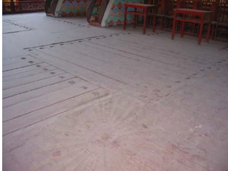
Pic. 7. Large dijing in the middle of the floor of the Longevity Stage. Photo taken inside the Longevity Stage of the Pleasant Sound Pavilion by Sasiporn Petcharapiruch on November 11, 2004.
