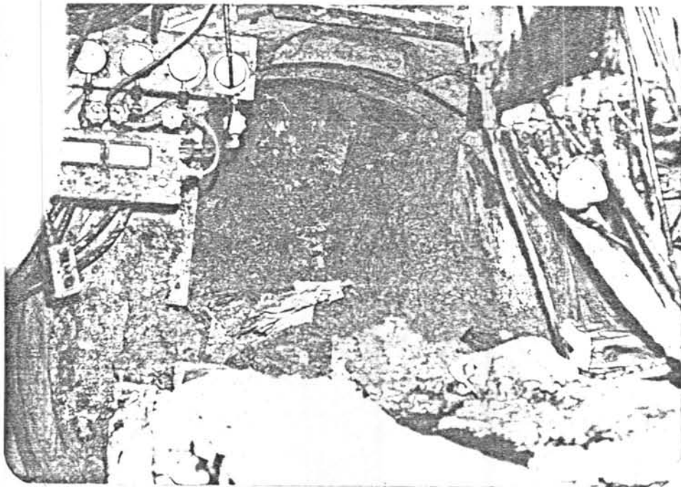
Fig. 71 The failure of tunnel face from the unsuitable tunnelling machine
