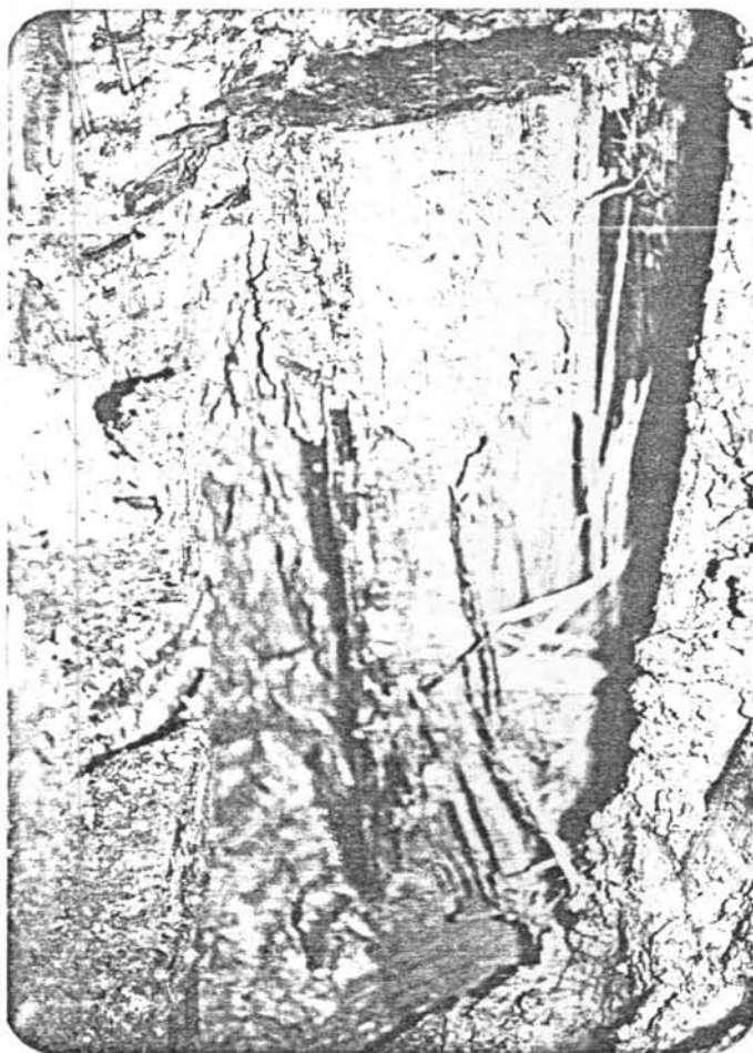
Fig. 71 The failure of tunnel face from the unsuitable tunnelling machine
