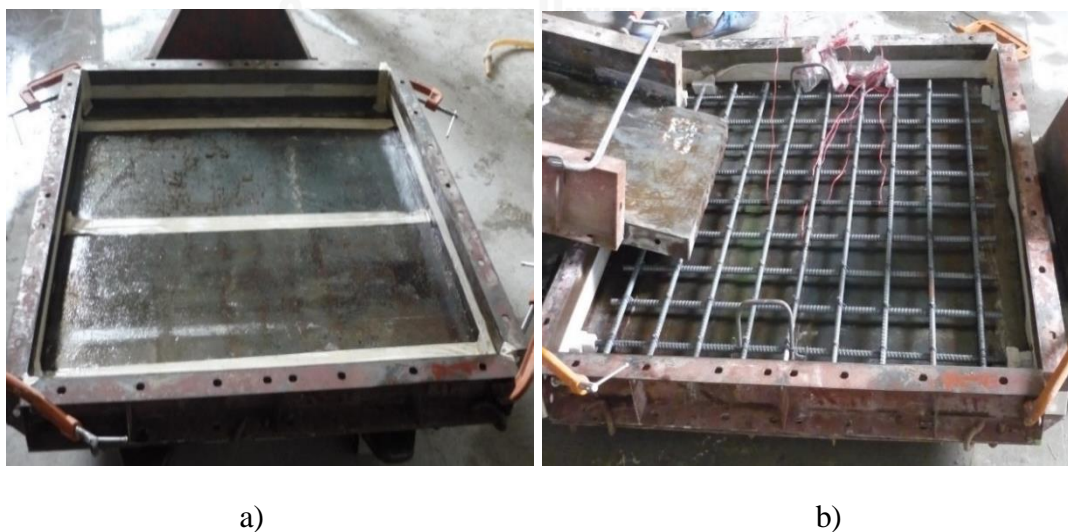
Figure 3.7 Slab formwork a) without rebar b) with rebar
