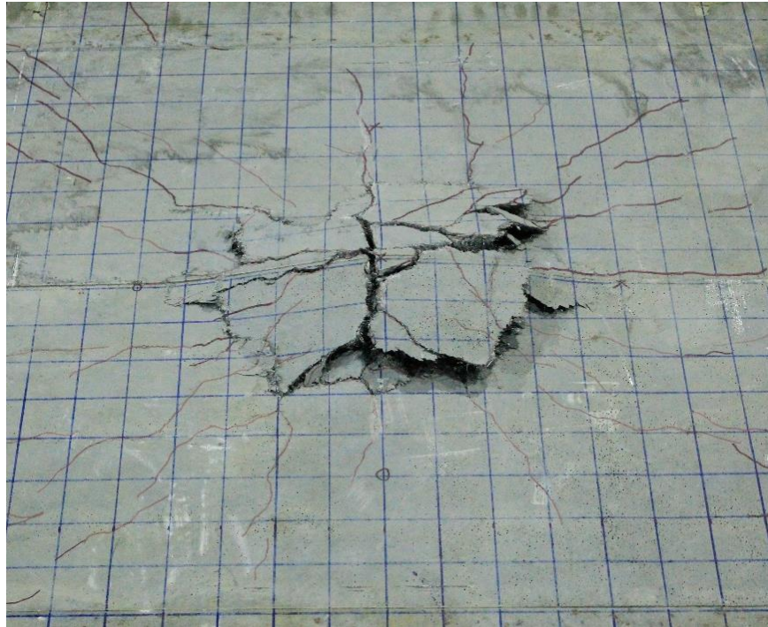
Fig A7 - Failure surface of the slab S07
