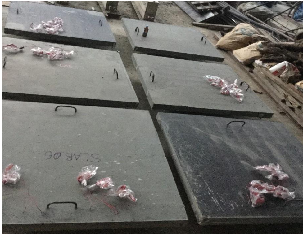
Figure 3.11 UHPFRC slabs after removing the mold
