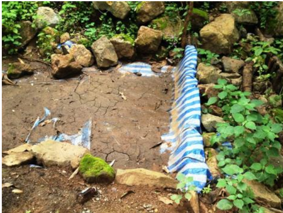
Figure AP-6 The monitoring check dam near the agricultural area at OB_SED 10
