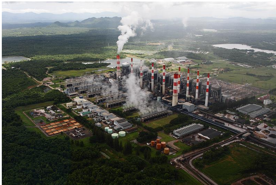
Figure 15 Mae Moh EGAT, Lampang lignite power plant (M. M. EGAT, 2012)
