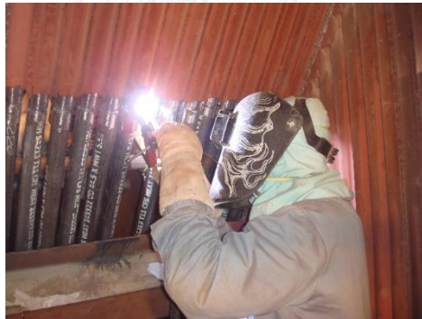
Figure 10 Welder is welding the pipe at Mae Moh powerplant
