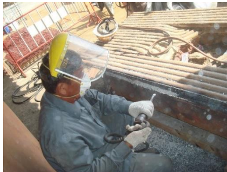
Figure 11 Turner is compound the pipe at Mae Moh powerplant
