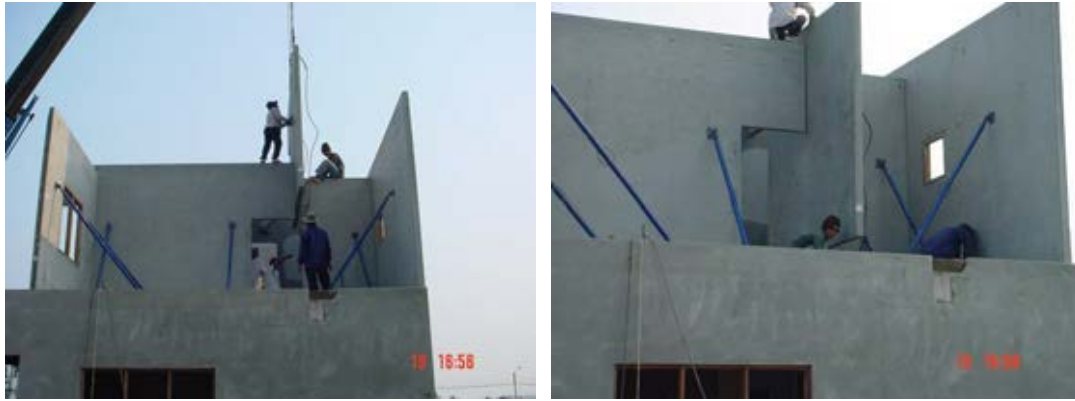
Figure 4.17 Installation between prefabricated members
