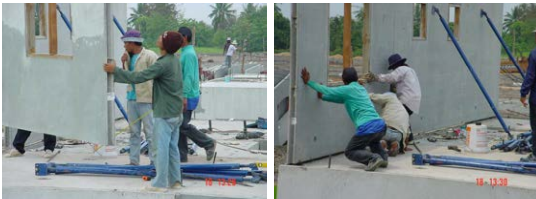
Figure 5.18 Erectors handle a prefabricated member at the location
