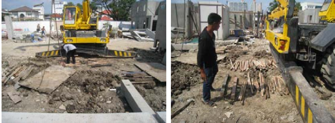
Figure 7.49 Operator applied another material for the machine set up
