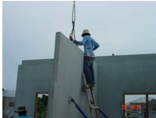
Figure 5.28 Unhook a prefabricated member
