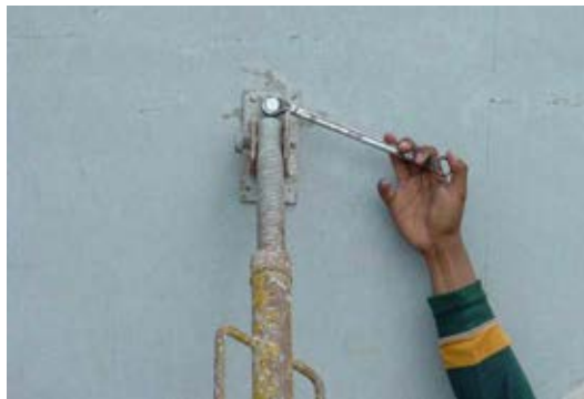
Figure 5.22 Fastening a bolt
