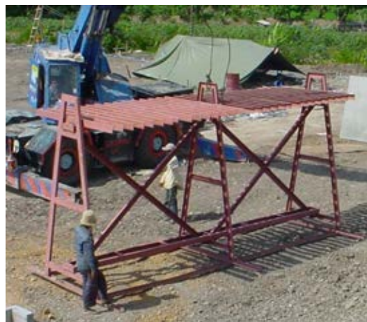
Figure 6.7 Stock rack at the construction site
