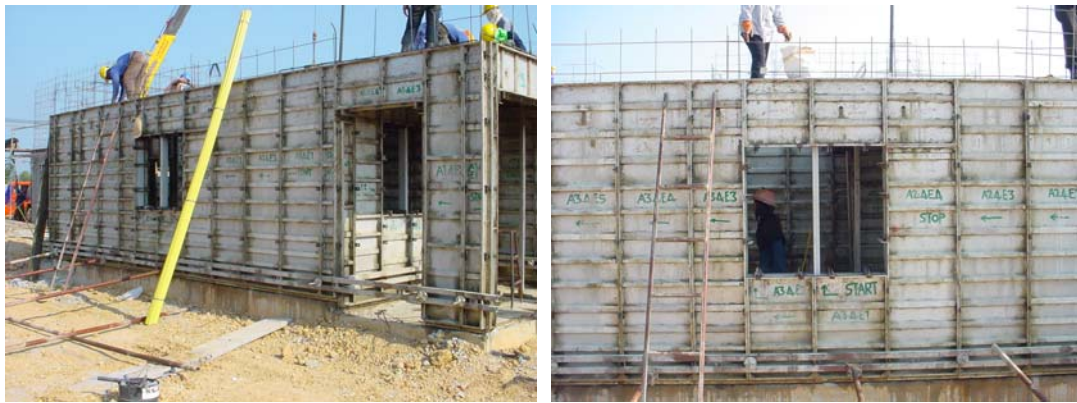
Figure 8.1 Formwork installation
