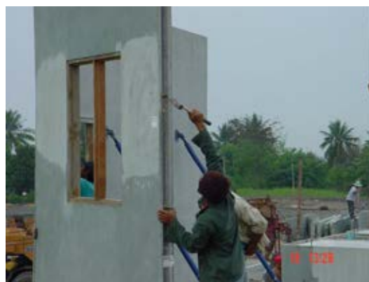
Figure 5.19 Erectors bend the steel loops
