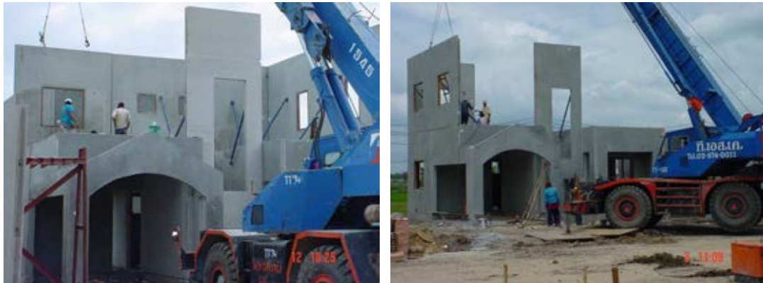
Figure 4.15 Different installation sequences
