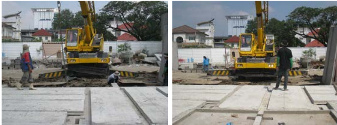
Figure 5.39 Support work from workers
