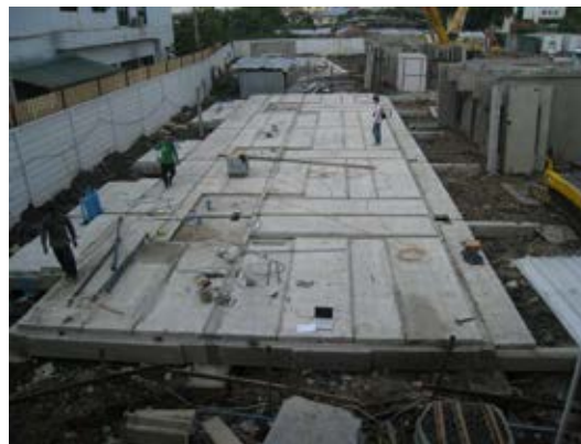
Figure 7.41 The eleventh block before the installation process
