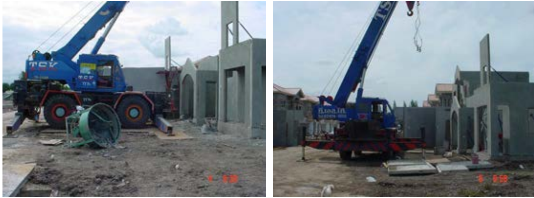
Figure 4.26 Different alignments of mobile crane
