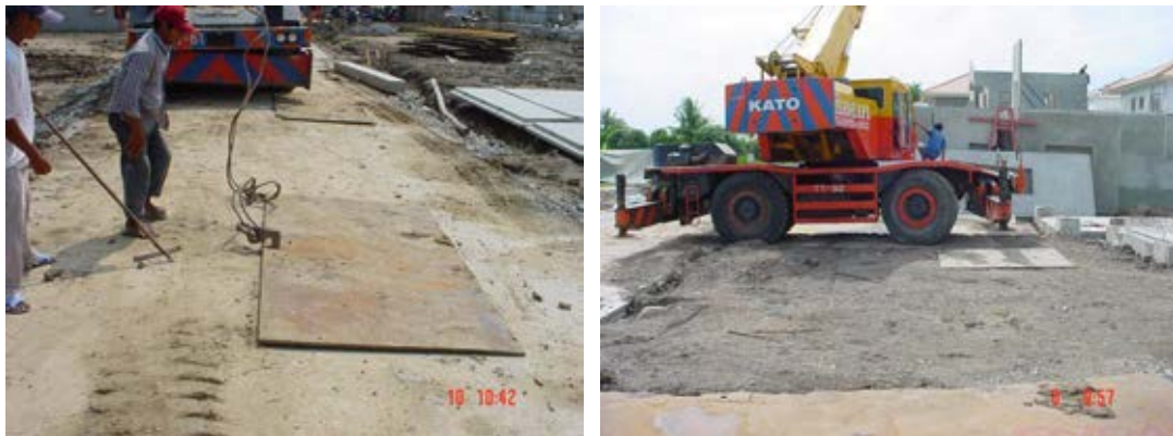
Figure 4.27 Set up the mobile crane and support from workers
