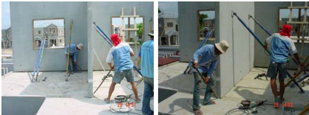
Figure 5.26 Alignment adjustment
