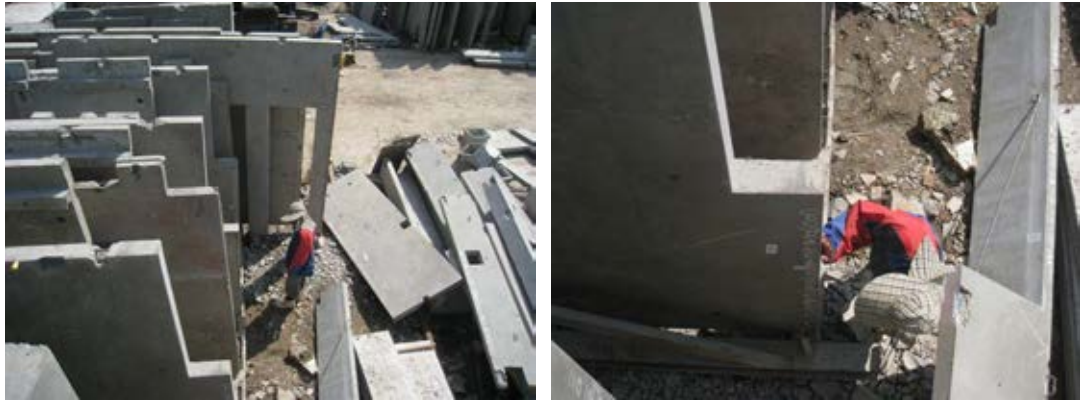
Figure 5.15 Stockman finds a prefabricated member
