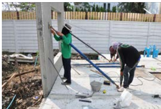
Figure 7.54 Erectors temporary shored the prefabricated member
