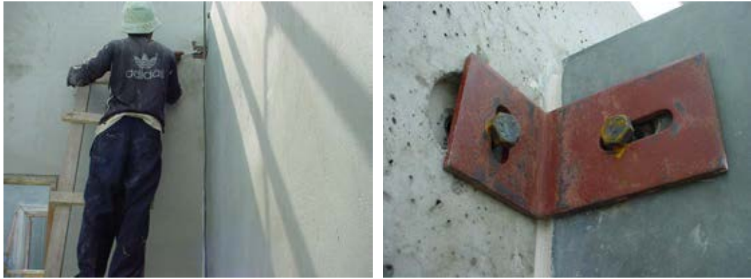
Figure 4.6 Bolt fastening joint
