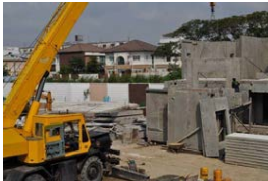
Figure 7.52 Mobile crane lifted a member
