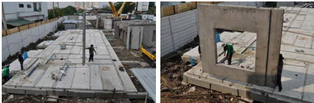
Figure 7.53 Prefabricated member was lifted and installed
