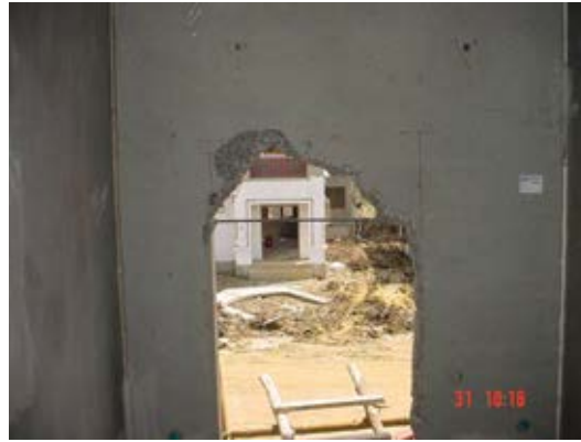
Figure 4.37 The mistake from manufacturing process
