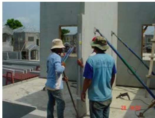
Figure 5.27 Measurement in the adjustment action
