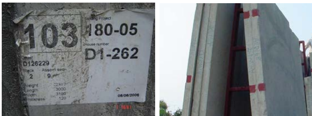
Figure 4.11 Prefabricated member marking
