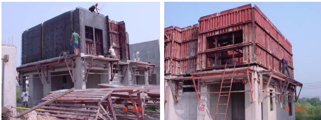
Figure 8.2 Formwork installation
