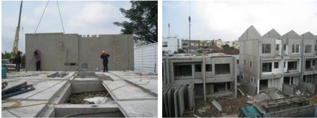
Figure 7.39 The overview of the prefabricated structure
