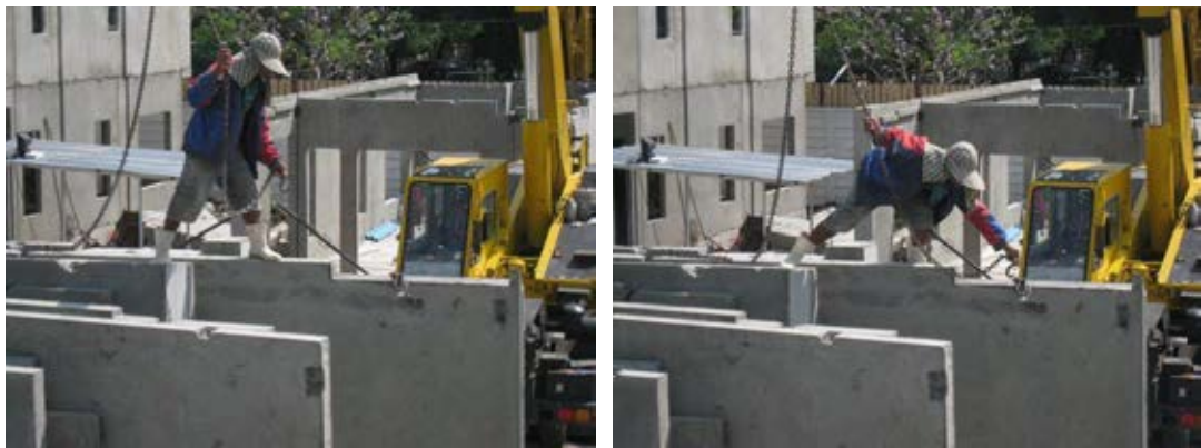
Figure 5.16 Stockman hooks a prefabricated member
