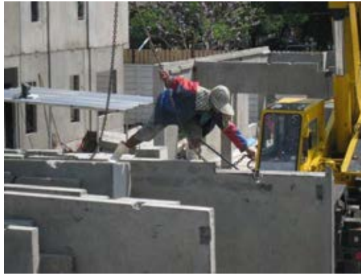
Figure 7.51 Stockman hooked a member
