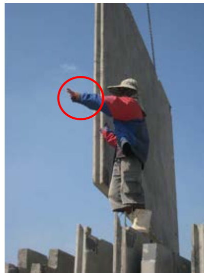
Figure 5.17 Stockman communicates with the mobile crane operator
