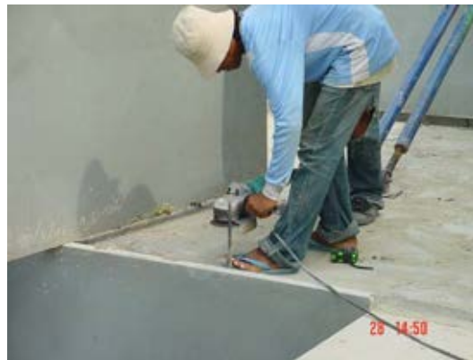
Figure 4.38 Dowel correction
