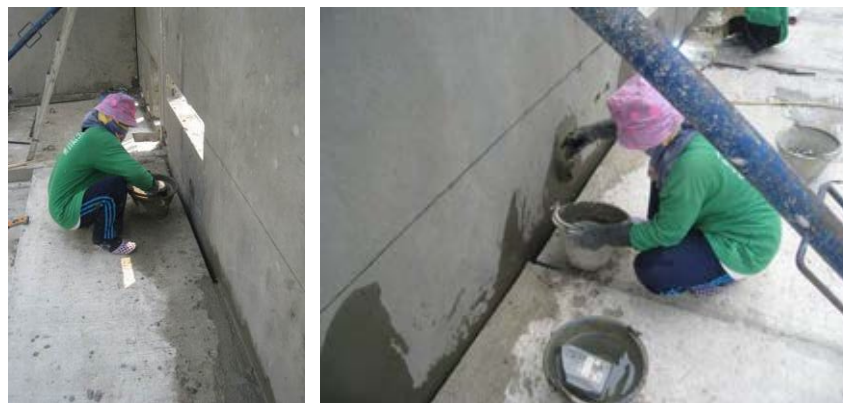
Figure 4.4 Wet joint
