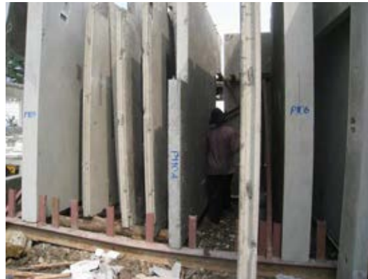
Figure 7.55 Prefabricated member marking
