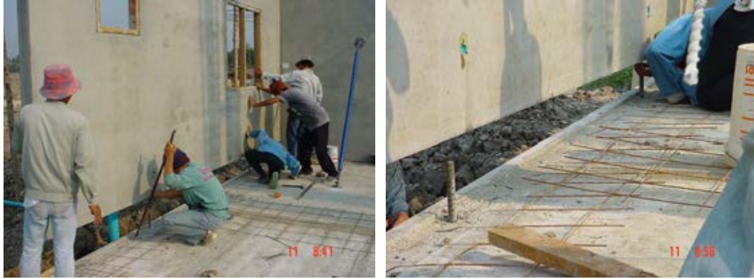
Figure 5.20 Two dowels must be inserted in the two dowel sleeves
