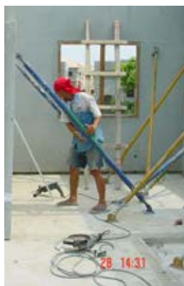
Figure 5.24 Inclination adjustment
