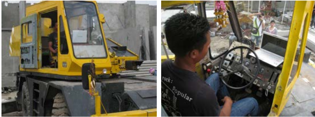
Figure 7.58 Laptop computer in the mobile crane cabin
