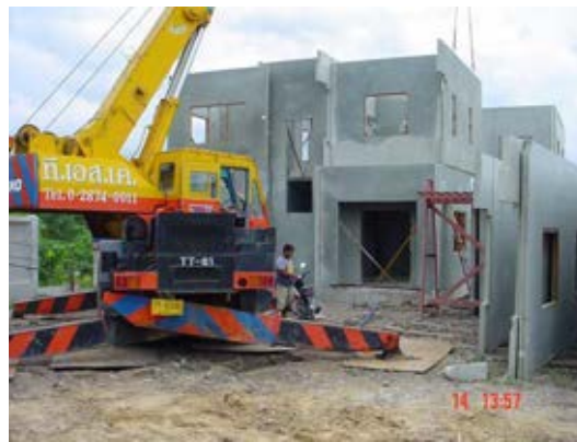
Figure 4.7 Prefabricated member lifting, moving, and installation
