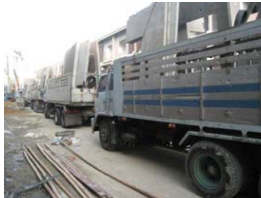
Figure 4.34 Order of delivery trucks at a construction site
