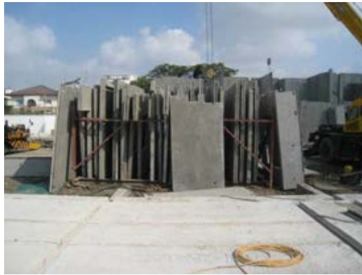
Figure 7.45 Overview of prefabricated members in a rack
