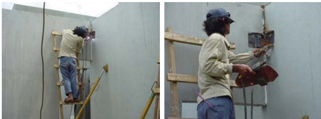
Figure 4.5 Weld joint
