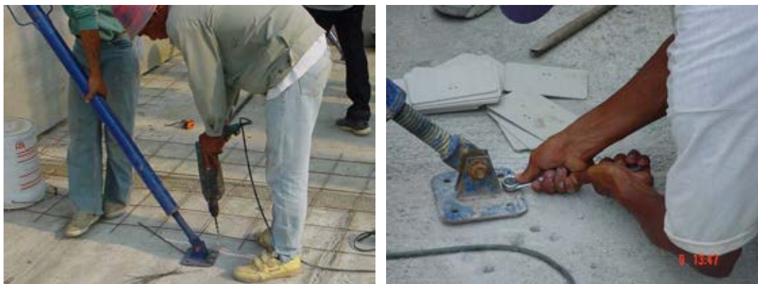
Figure 5.23 The use of bolt, prop, wrench, and drill for shoring
