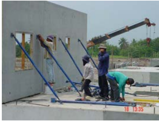
Figure 5.21 Shoring a prefabricated member
