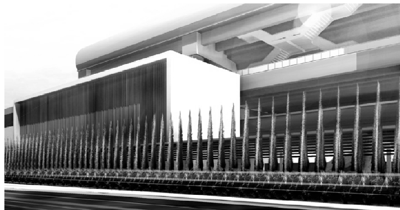
Figure 7.47 East station entrance and motorcycle parking
