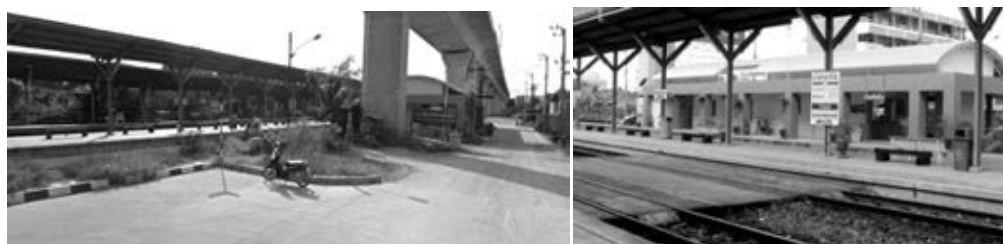
Figure 4.30 Ban Tap Chang train station
