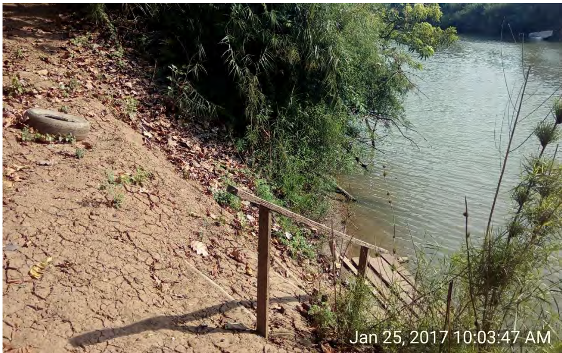
Figure 11. Bank slope near the borehole BC1 location.
