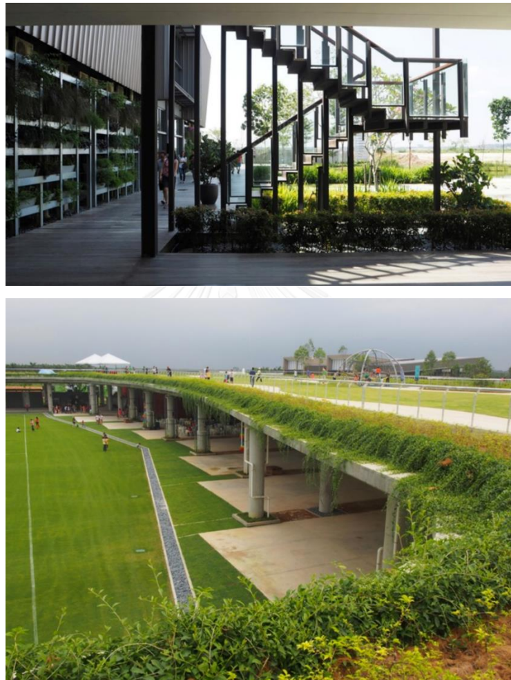
Figure47: The elevated play area, THE ARC at Bandar Rimbayu. Source: Steven Ngu & Andy Lim, 2016
