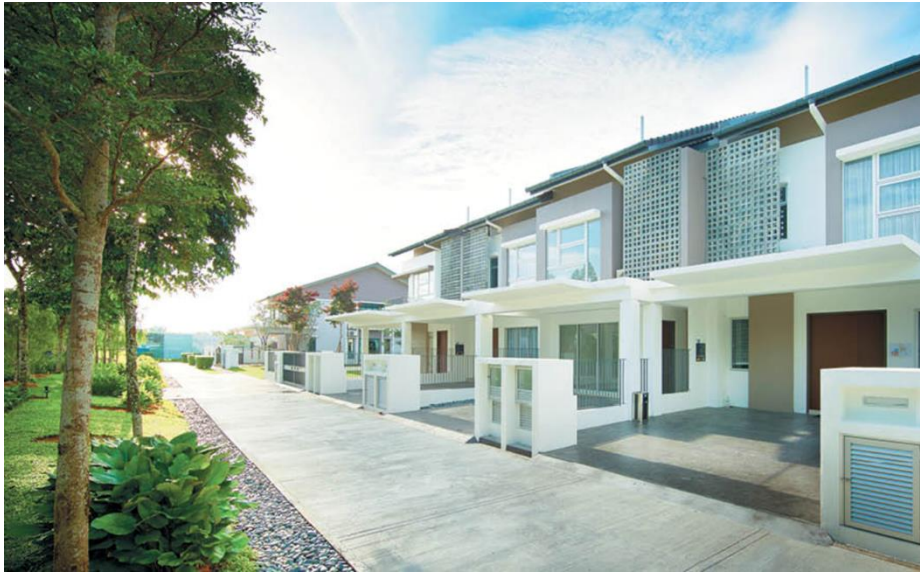
Figure52: Penduline Residence frontage.
