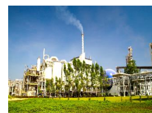
(c) Chemical Recovery for Plant I
