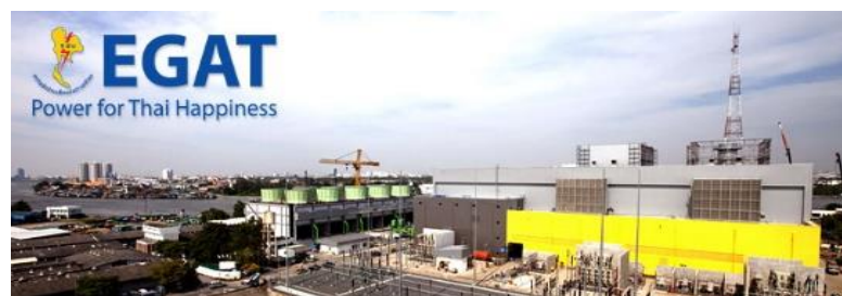
Figure 20: Electricity Generating Authority of Thailand (EGAT)
