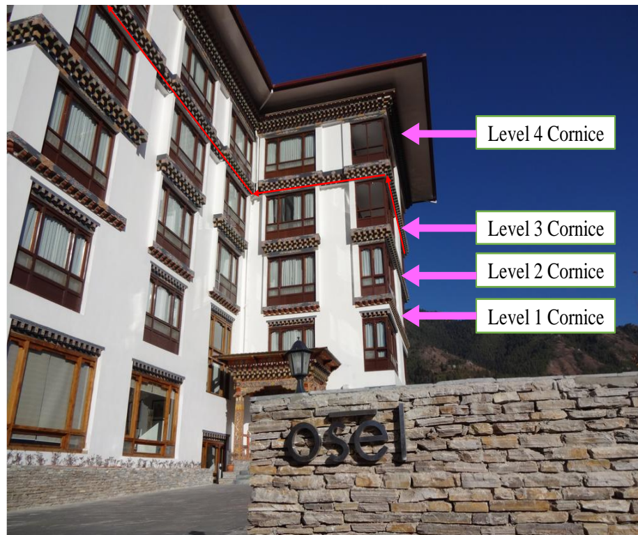
Figure 2-6 Five story modern building with cornice projection ( http://www.oselbhutan.com )
