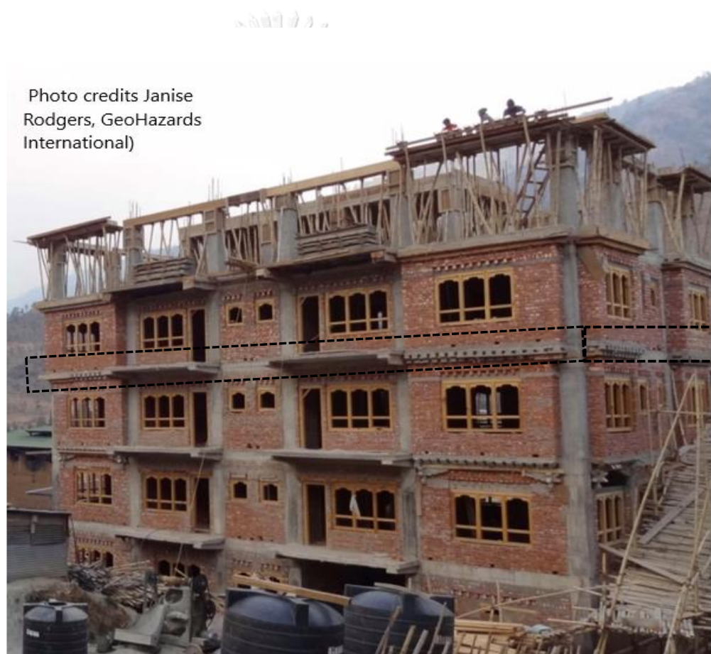
Figure 2-5 Modern building during construction
