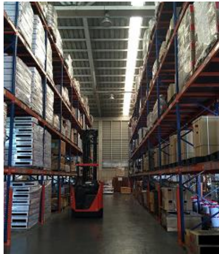
Figure 3.30: Single-deep Selective Rack Area of Warehouse 8
