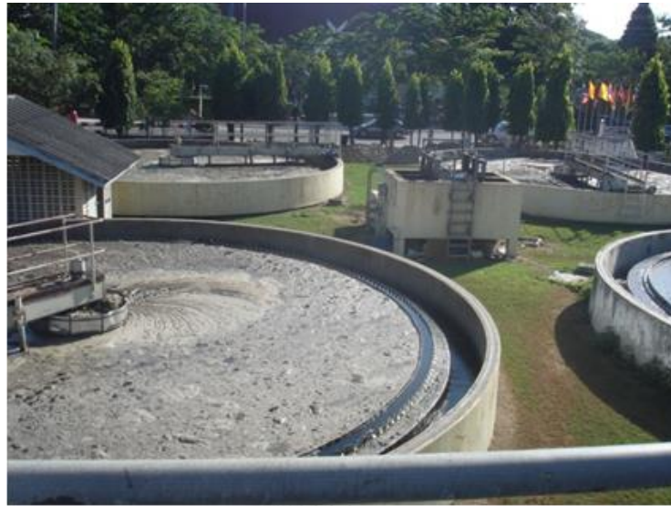
Figure 3.1 Domestic wastewater treatment plant at Chiang Mai University
