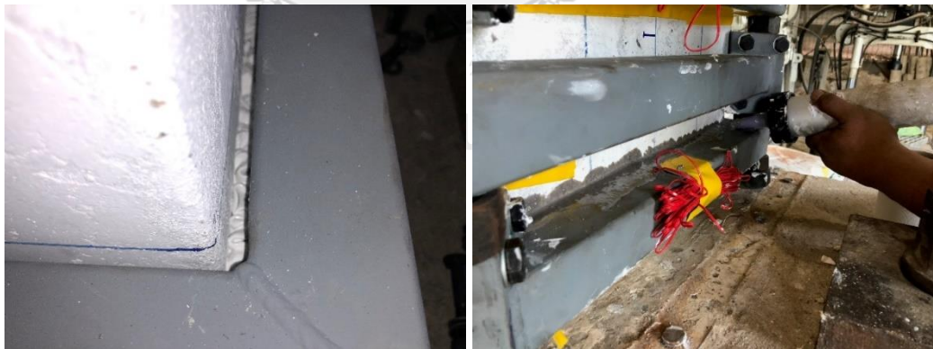
Figure 5.15 Gap-fill between column and steel collars by using epoxy
