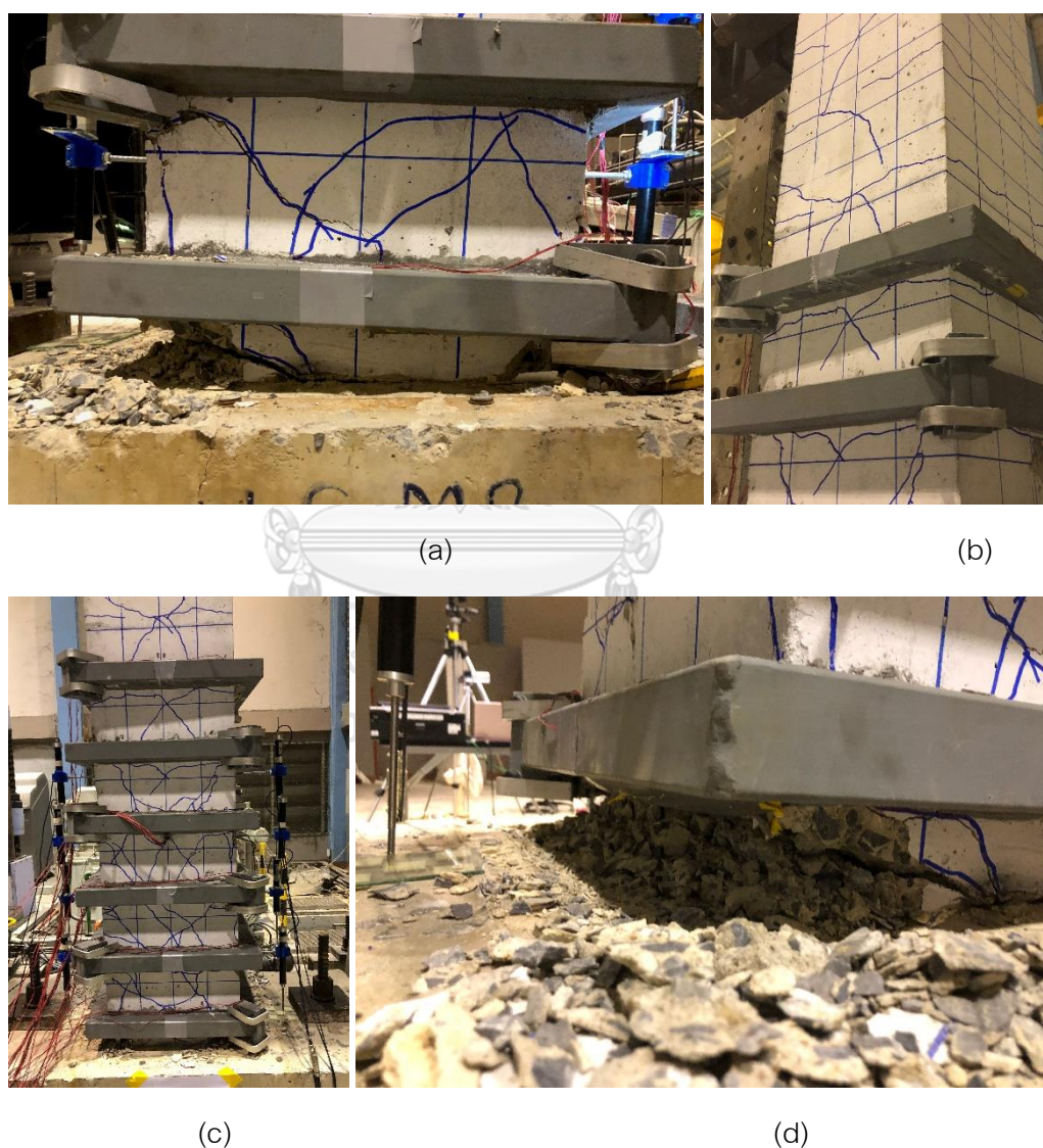
Figure 5.24 Flexural joint failure of strengthening lap-splice column SC2
