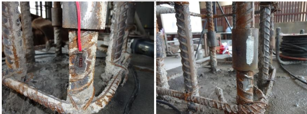
Figure 3.10 Strains measurement of reinforcing steel and mechanical splice
