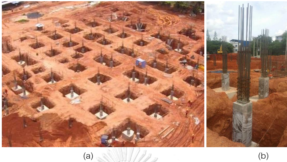
Figure 1.3 (a) Construction practices in the building structures in Thailand (b) The longitudinal reinforcement for lap splice steel bars to the next floor.
