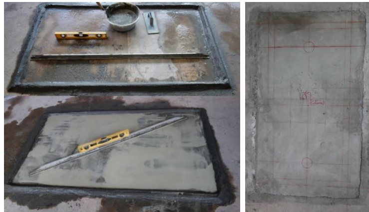
Figure 3.3 Prepare ground level and grid line for construction
