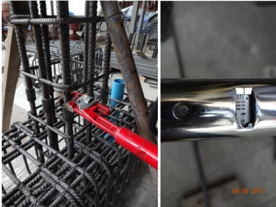
Figure 3.7 Initial torque of the threaded collars of approximately 200 N-m.
