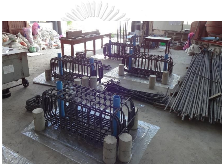
Figure 3.4 Rigid footing reinforcement detailing
