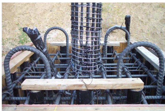
Figure 2.13 Column with Threaded Bar Couplers [23]
