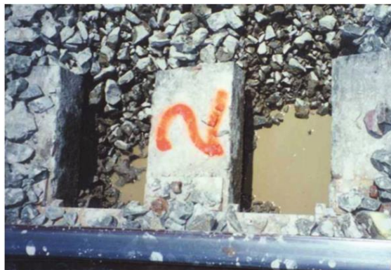
Figure 2.2 Ponding water in ballast layer (Indraratna et al., 2011)
