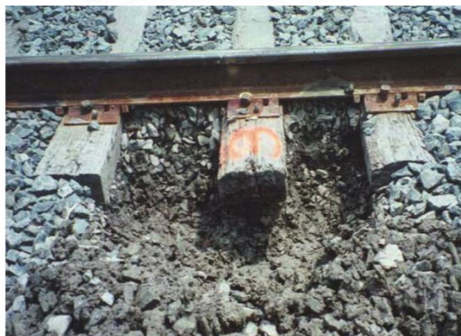
Figure 2.1 Fouling of ballast (Indraratna et al., 2011)
