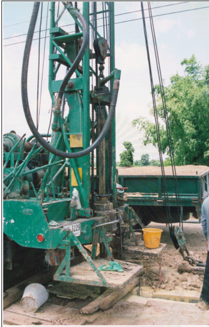
Figure1.12 The drilling rig in the study area.
