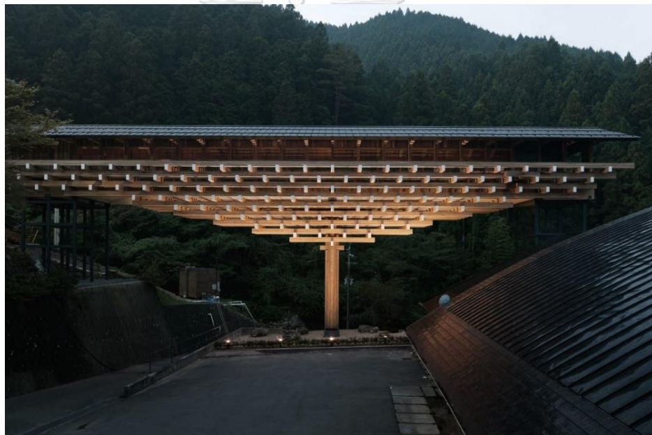
Figure 61: Yushuhara Bridge Museum (Source- www.archdaily.com )
