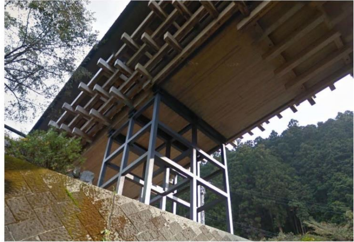
Figure 63: Construction joint between wood and steel structure (Edited the source-Kengo Kuma's official website)
