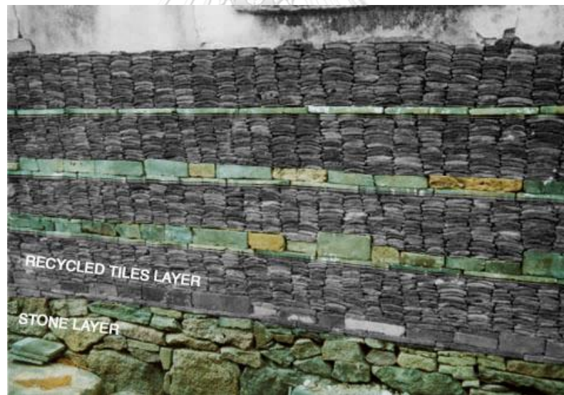
Figure 51: Traditional Wapan Construction Technique (source- http://www.zhxxww.net )
