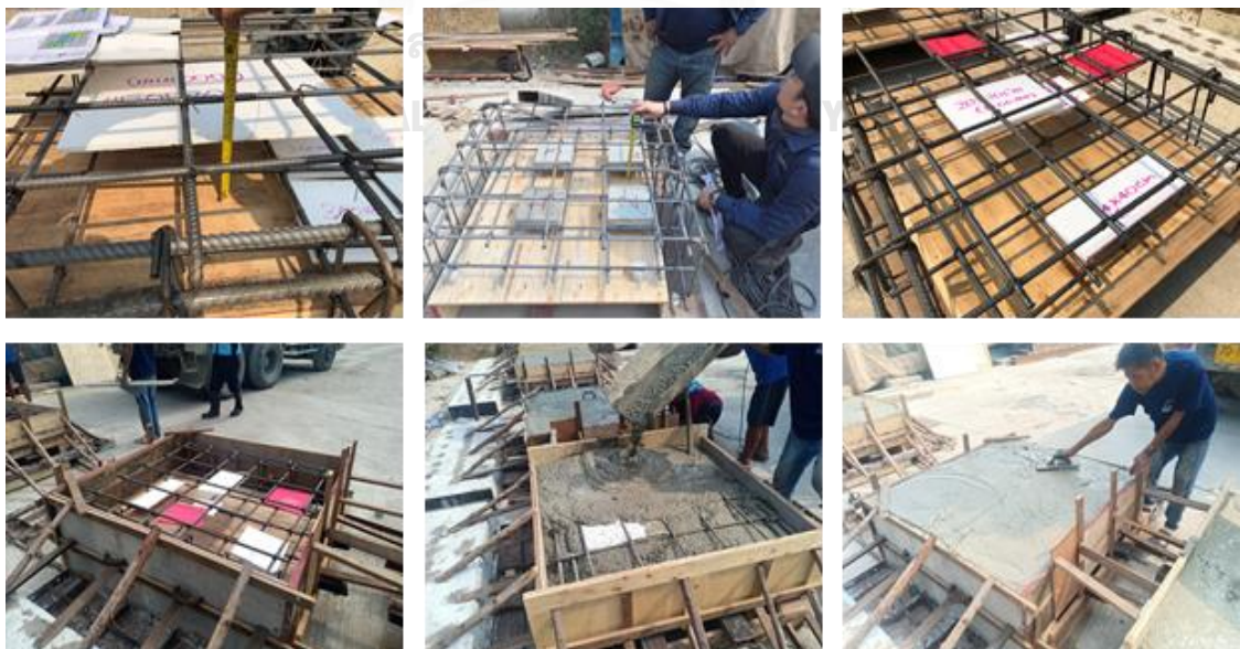
Figure 23. Totally four RC mock-ups with simulated defects were constructed.
