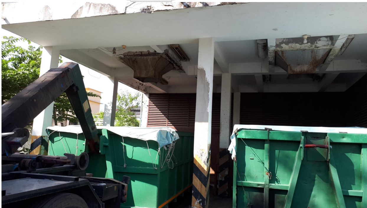
Figure E8 Sludge storage at WWTP B.
