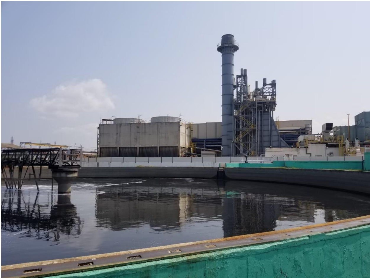
Figure E4 Sedimentation tank at WWTP A.
