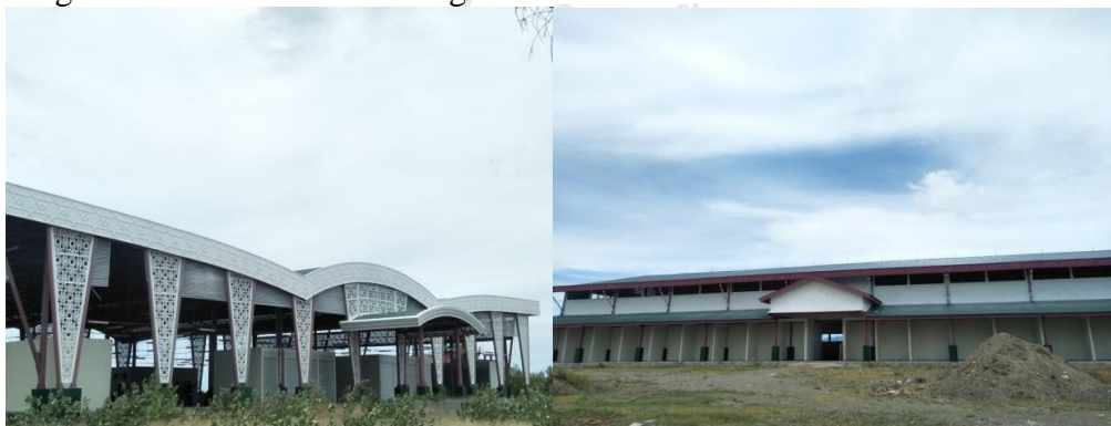
Figure 8. Fish market building
