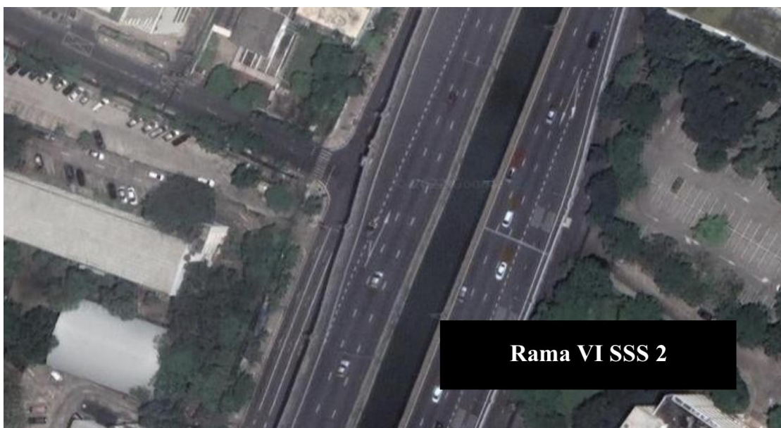
Figure 4-23 Satellite view of Rama VI SSS 2 intersection.
