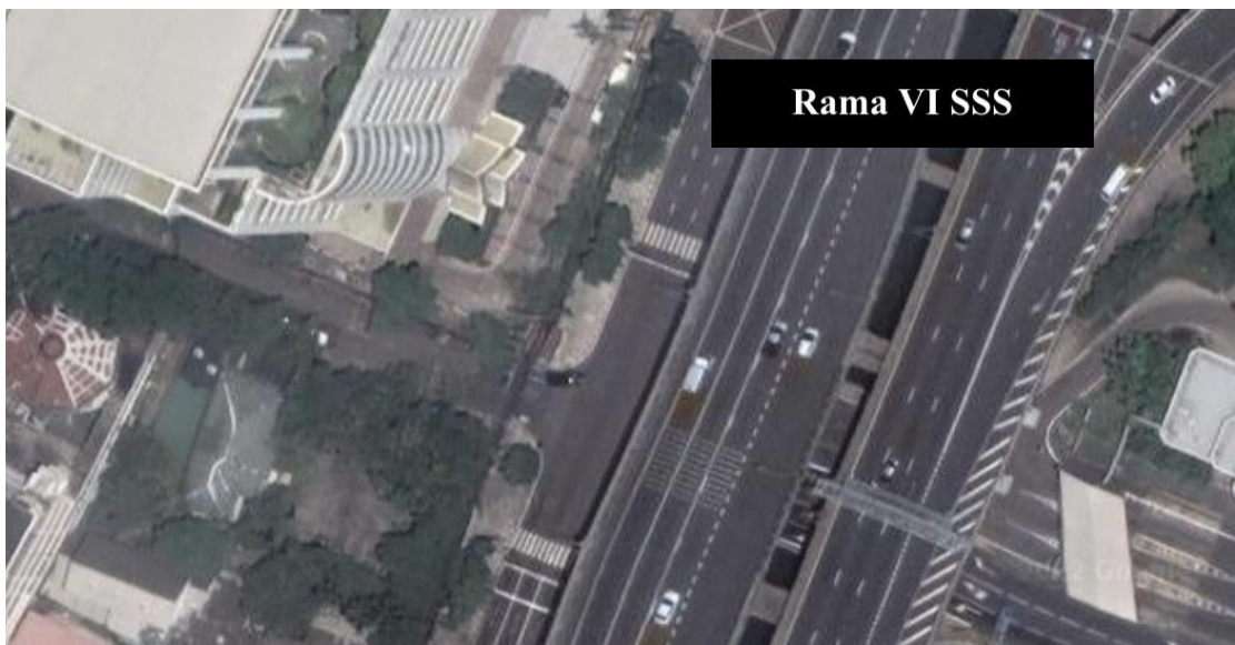
Figure 4-24 Satellite view of Rama VI SSS intersection.
