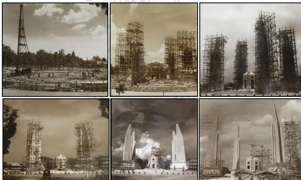
Photo 20. The pictures of the Democracy Monument construction.
